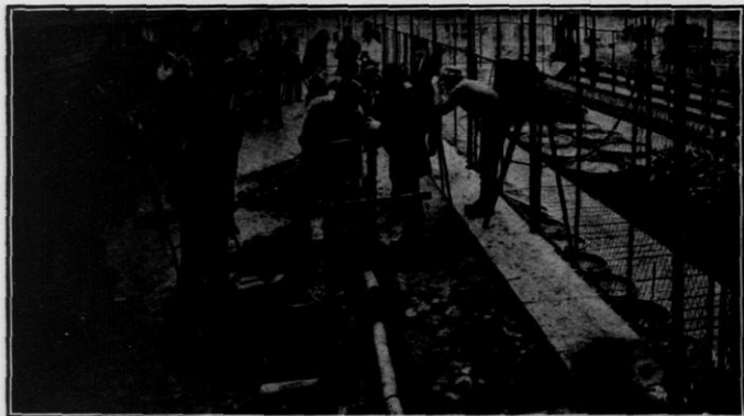
Land drainage is of paramount importance in Wisconsin and students in the Short Course are given practical work in laying tile.
