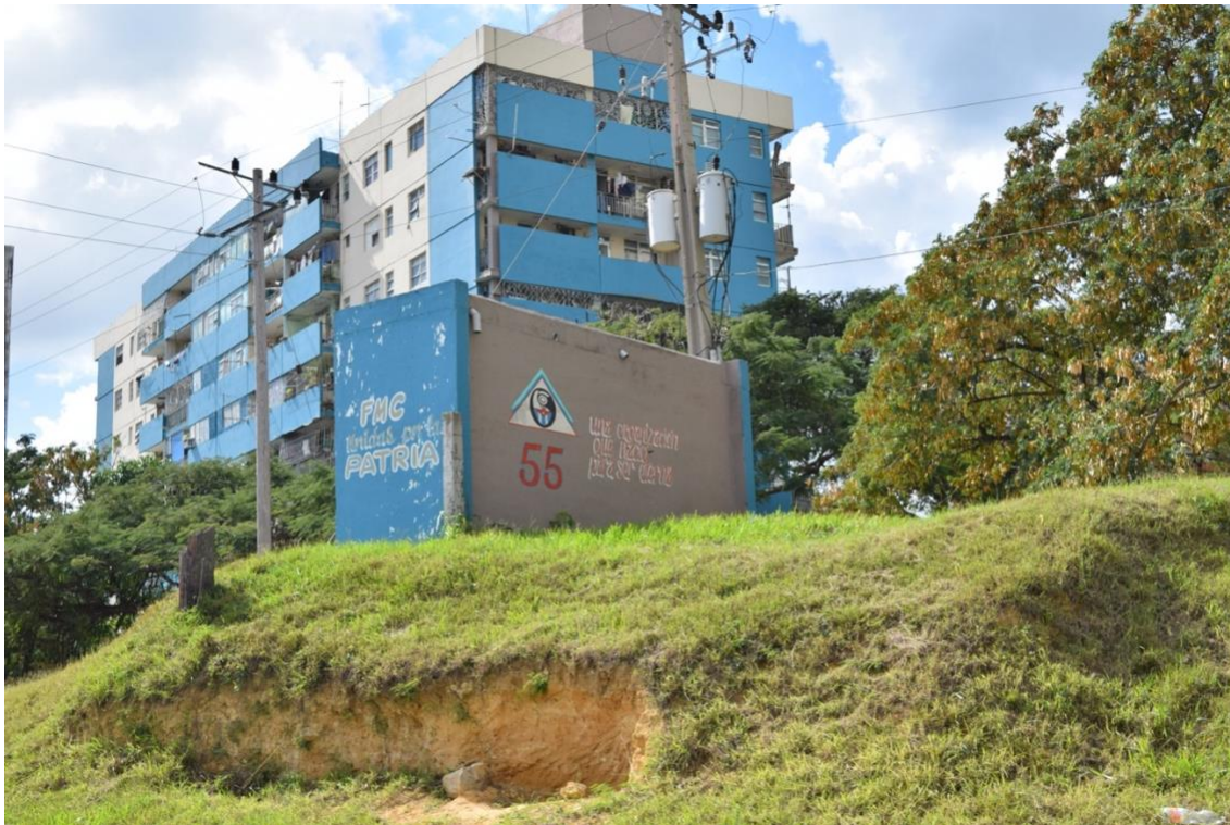
Photograph taken by author in January 2016 of a microbrigade building in the city of Cienfuegos.
