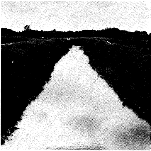
FIGURE 7. Goose Lake Canal, a channelized stream in southeastern Wisconsin. Note the lack of heterogeneity in flow patterns in the channel and the absence of in-stream and bankside cover. (Photo by Paul Kanehl.)
