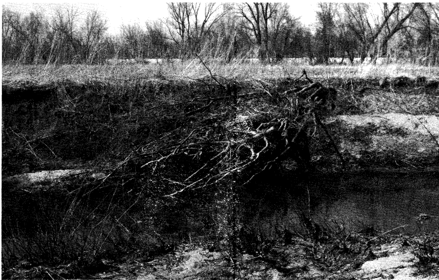
FIGURE 4. A tree revetment in Court Creek in west-central Illinois, installed using the George Palmiter river restoration techniques. The revetment has been damaged by ice and only partially protects the severely eroded bank. (Photo by John Lyons.)
