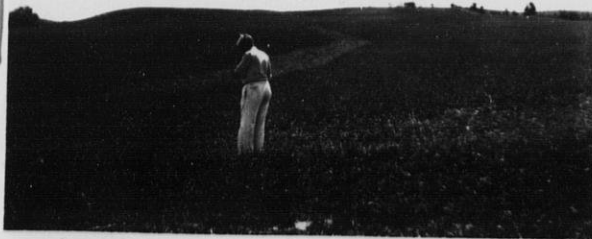
Permanent sod runs such as these are preventing formation of gullies. This sod run was constructed in the summer of 1939 on a demonstration farm in the town of Scandinavia, Waupaca County.
