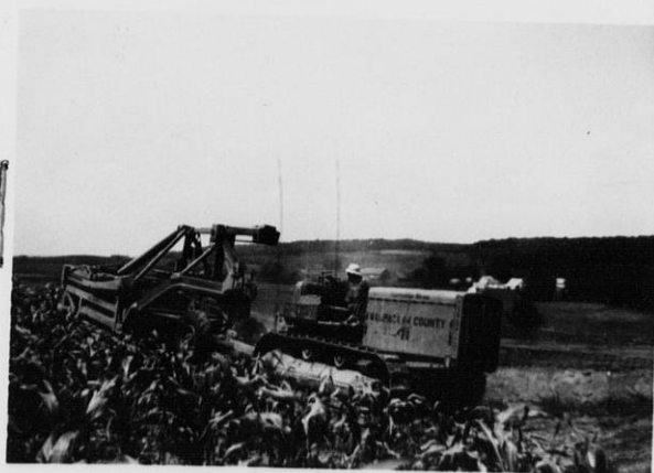
County power scraper in action on the dirt fill for the dam. This machine moved 500 yards of dirt in 7 hours at a cost of $52.00.
