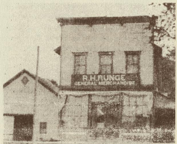
The old General Store on Howell Road
