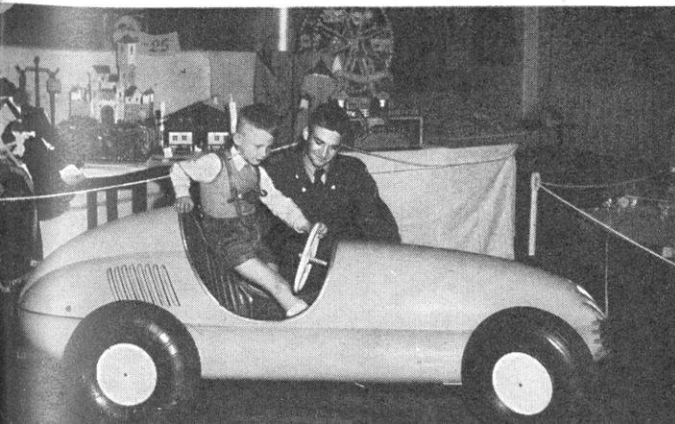
Miniature racer built by three teen-age Garmisch youths has two forward speeds, can travel 25 miles per hour.
