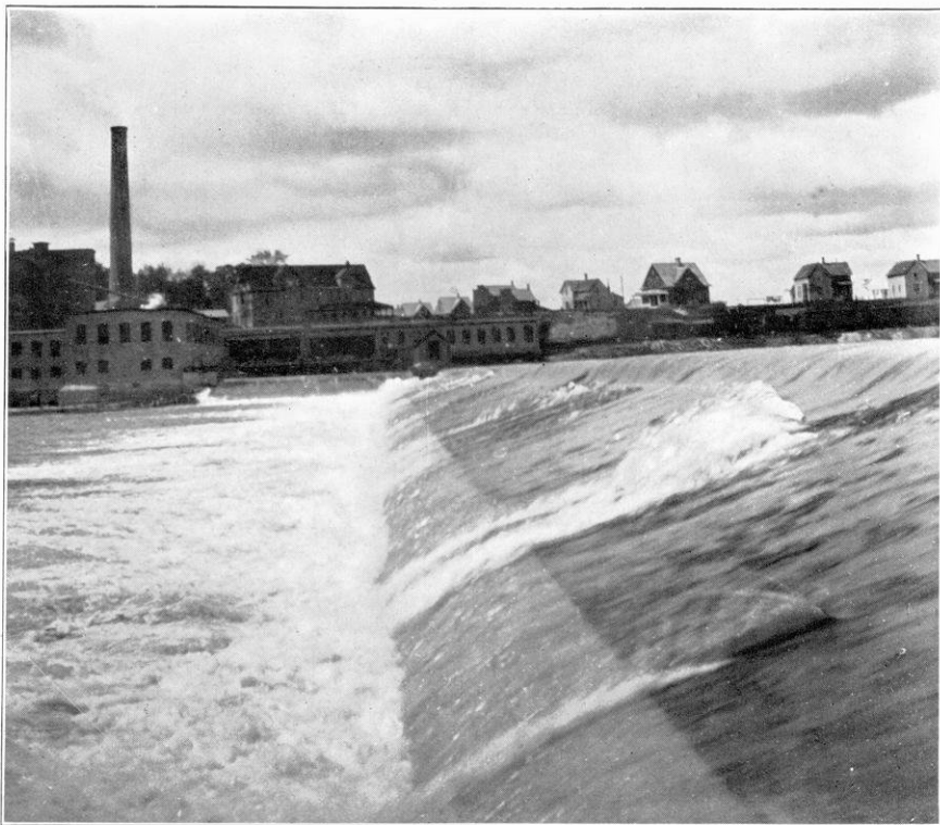
Fig. 1. U. S. DAM AT KIMBERLY, WISCONSIN, FOX RIVER. Head 9.7 feet.
