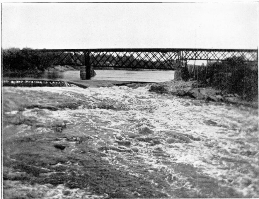
Fig. 1. DAM AT BLACK RIVER FALLS. PARTLY CARRIED AWAY BY HIGH WATER.
