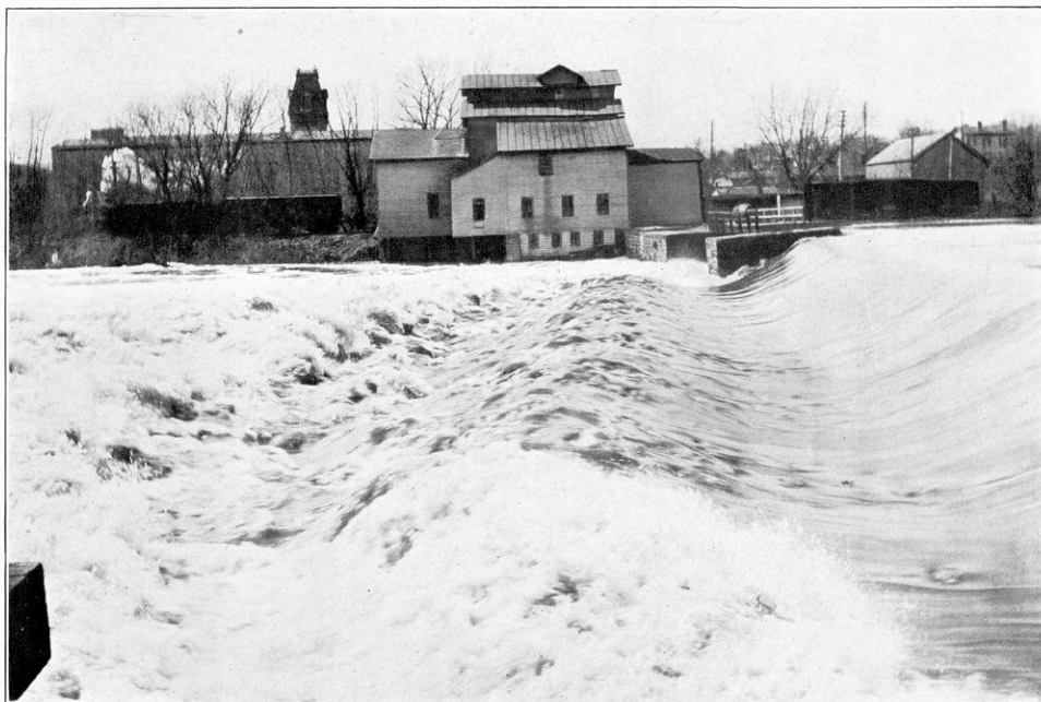
FORDS DAM. ROCK RIVER AT JANESVILLE. High water. Head, 8 feet.
