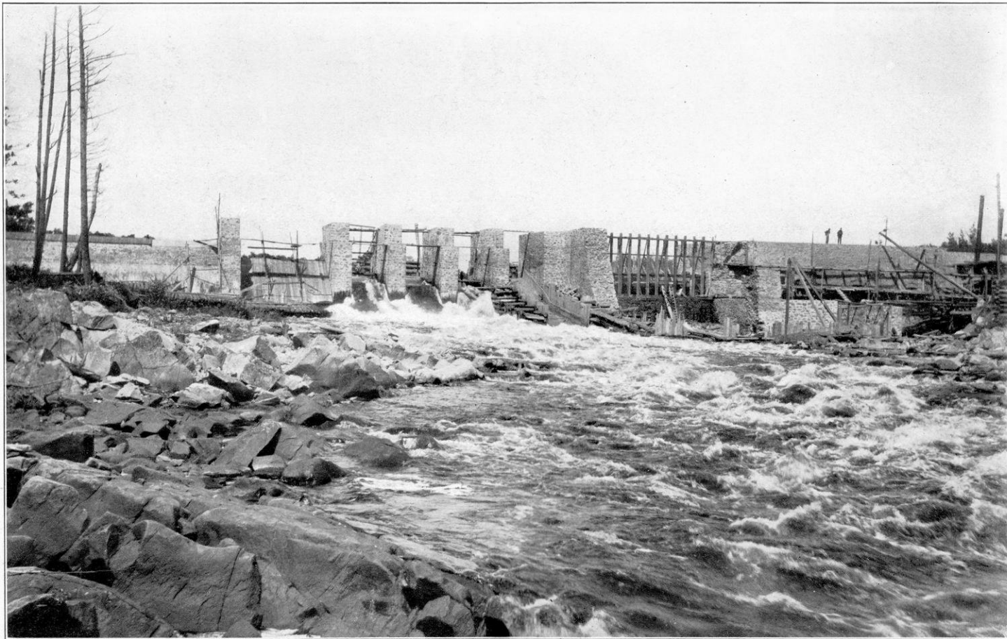
NEW DAM, COMPLETED 1907, DEVELOPING THE UPPER THIRD OF GRANDFATHER RAPIDS, WISCONSIN RIVER. Head about 31 feet.
