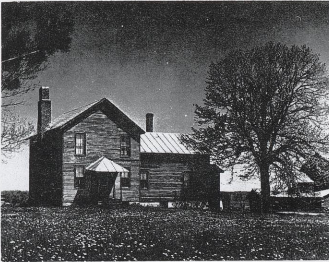
The buildings of the Fritz Hoffman farm, once known as one of the Consolidated Farms. This house was used as a boarding house.
