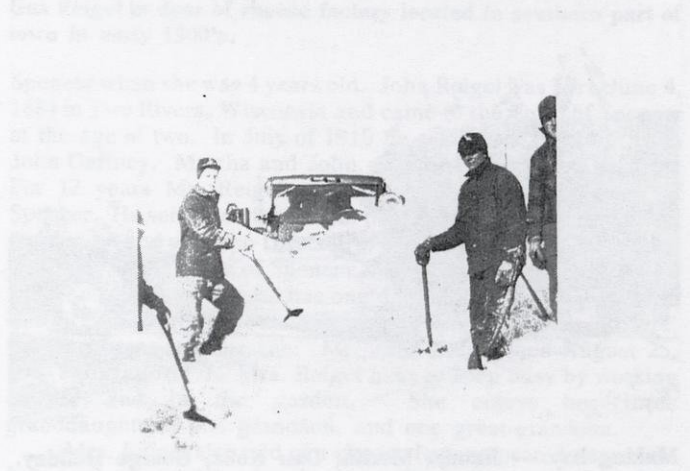
Lloyd Hoops, "Shorty" Hoff and Alvin Gauger, clearing the town roads.
