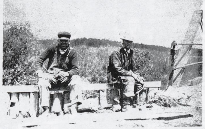
Contrasting yesteryear with today. Fred Foth and Frank Oelrich sit on the wooden portion of the bridge on County Trunk C which spans the Little Eau Pleine. Even the younger settlers of our town can remember when C was barely passable in the Spring.
