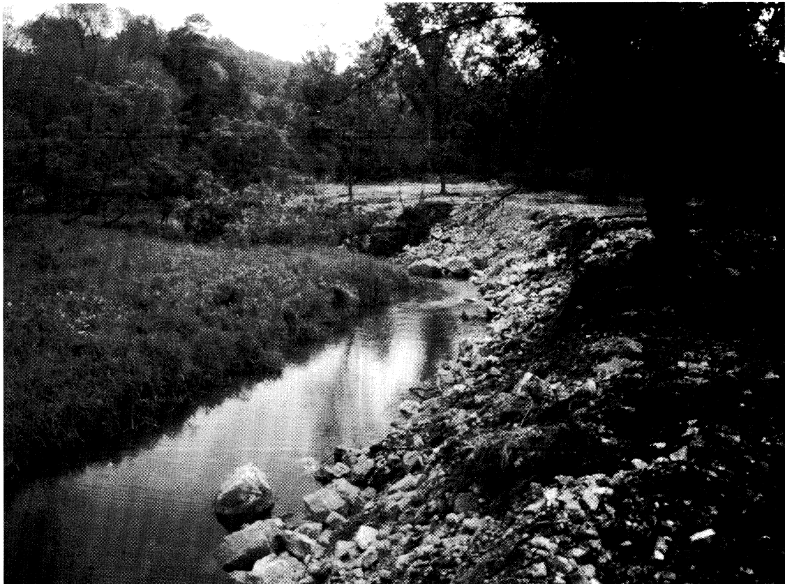
Figure 4. Intensive streambank riprapping stabilizes eroding streambanks, encourages downward streambed scour, and ultimately creates a deeper stream—Millville Creek, May 1991 (upper), and August 1990 (lower).
