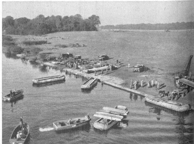
Preparation to throw pontoon bridge across river.
