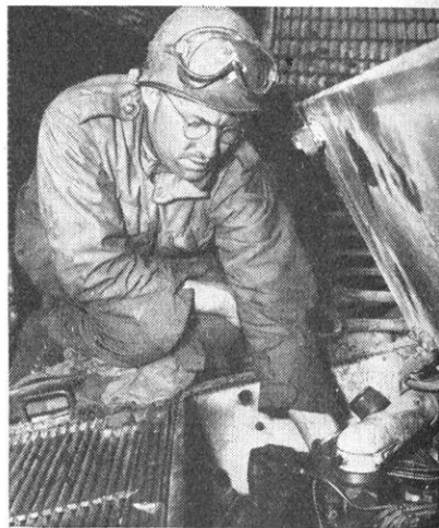
Making minor repairs.
