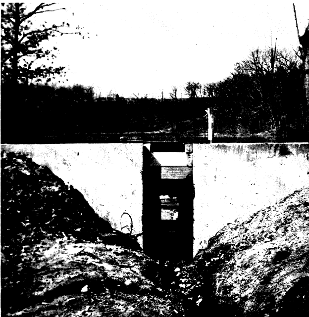
FIGURE 2. Concrete outlet structure at Pleasant Lake with the marsh in the background.
