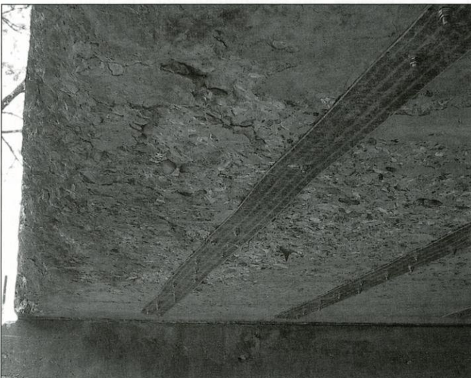
A view of polymer bandages on County Road 6120 in Phelps County, Missouri.
