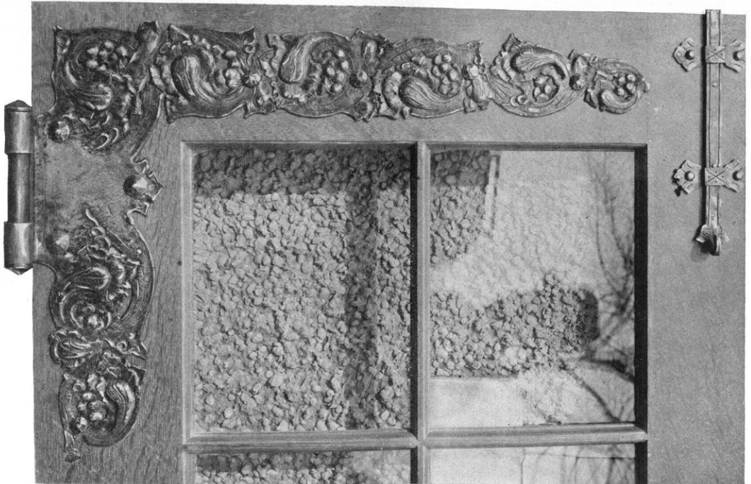
WROUGHT-IRON FITTINGS FOR A DOOR, HINGE AND BOLT, THE WORK OF MR. YELLIN.
