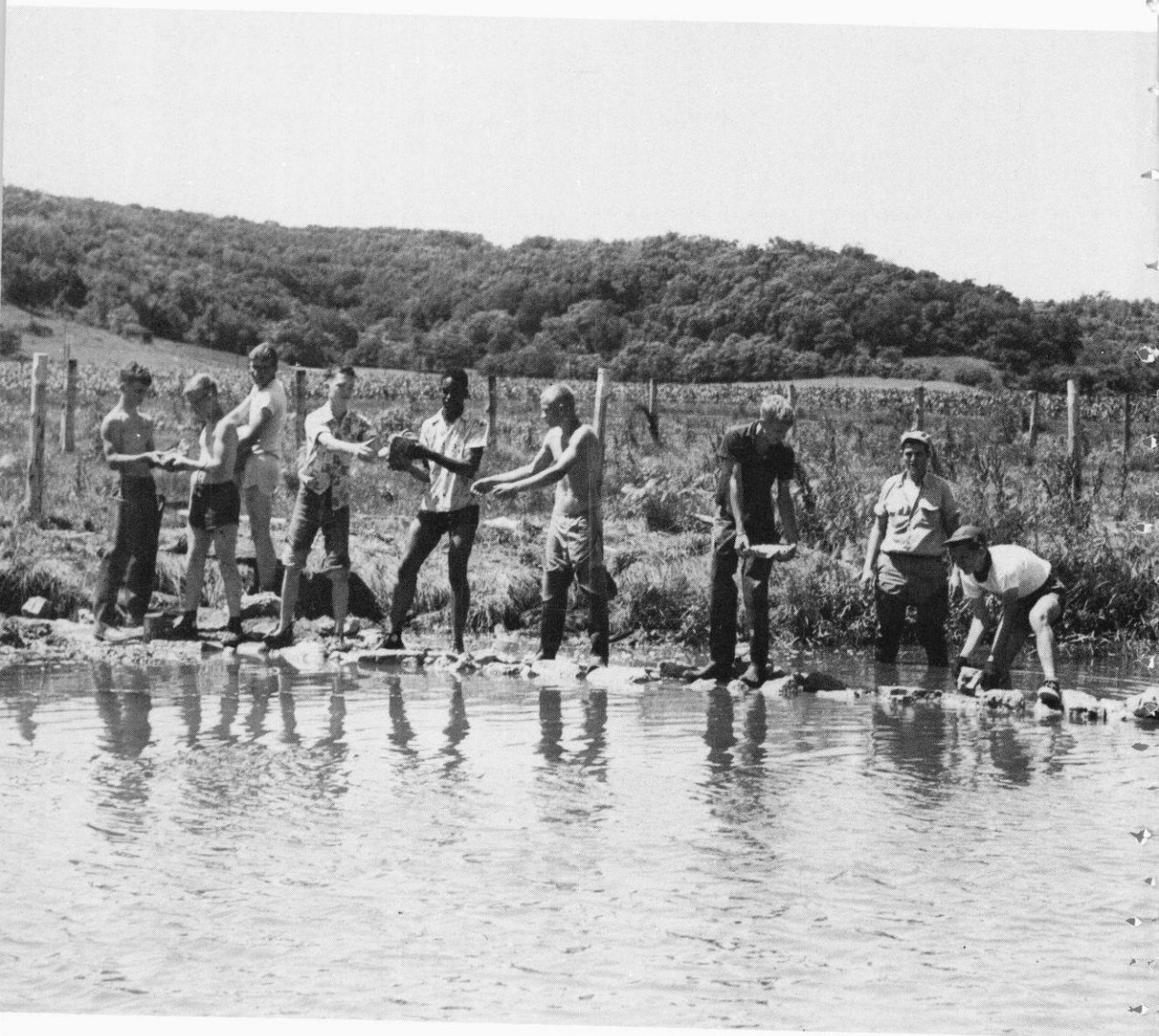
Boys in the summer conservation class build a rock deflector to increase the speed of the current.
