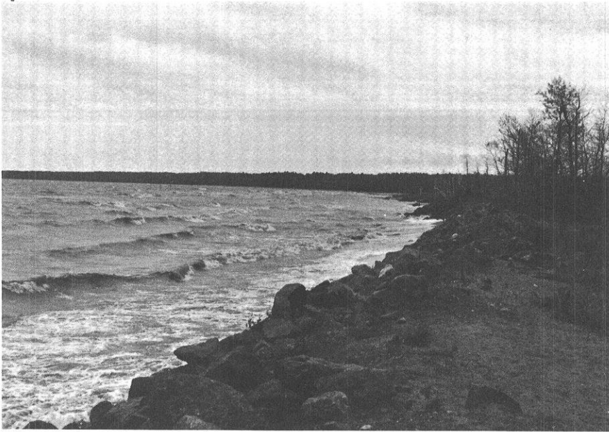
View of riprap along shoreline. Groins can be seen in distance.
