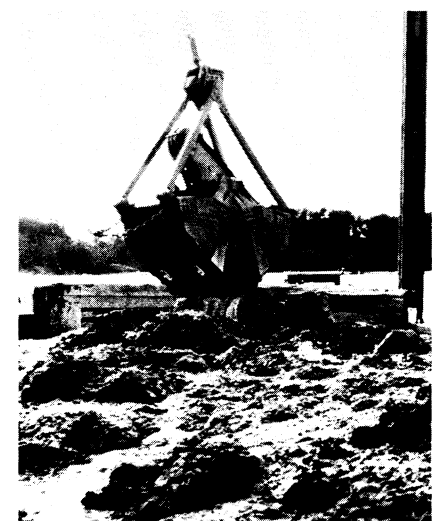
Some of the dredged material was too fine-grained for a beach nourishment project. This barge load was mostly clay and silt.
