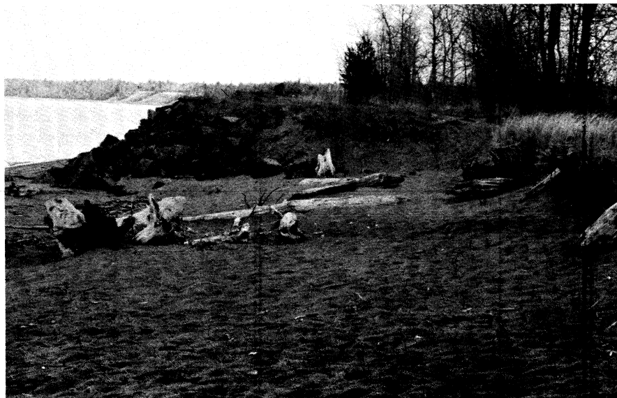
Beach berm erosion at the downdrift end of the riprap (May 1985).
