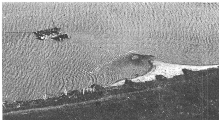
Littoral drift accumulated in front of the groins following the deposition of sediments.
