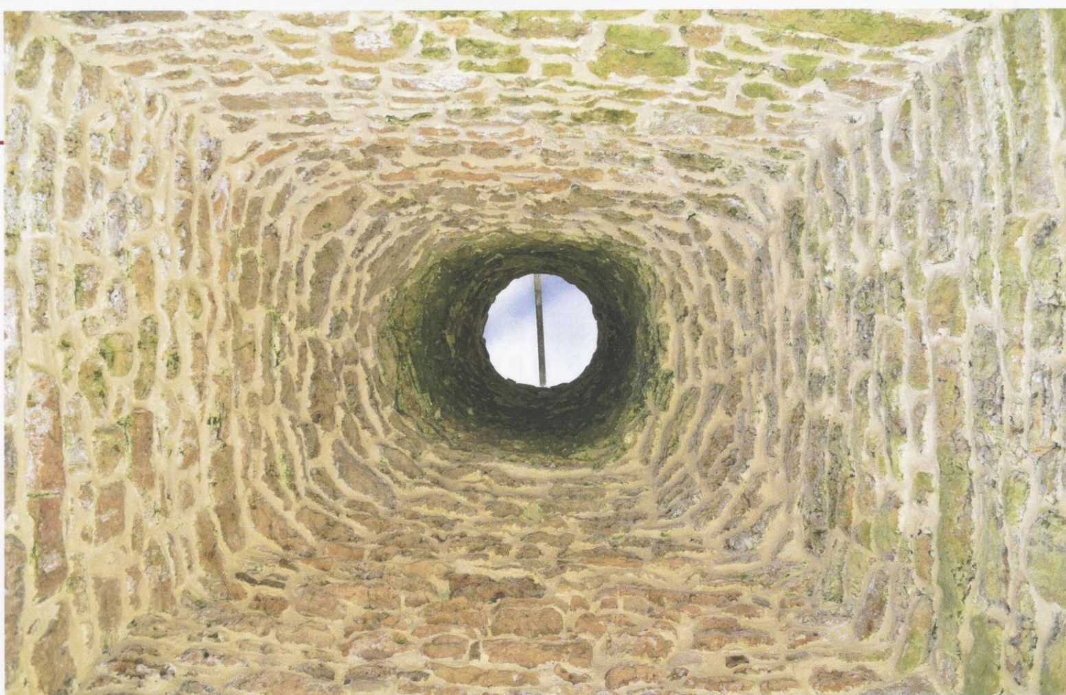
THE VIEW THROUGH A NOW ABANDONED MELTING FURNACE IN DODGEVILLE, WI. THE STONES LINING THE INSIDE OF THE STACK ARE STAINED GREEN FROM BOTH MOSS AND THE EFFECTS OF VAPORIZED METALS THAT WERE ONCE REFINED IN THIS FURNACE.
