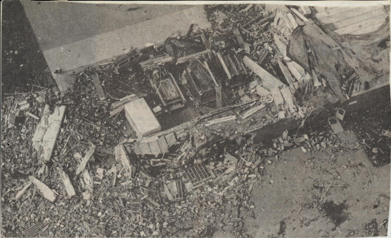
The blown-out wreckage of what used to be the Barneveld fire station looks like it was hit by a bomb.
