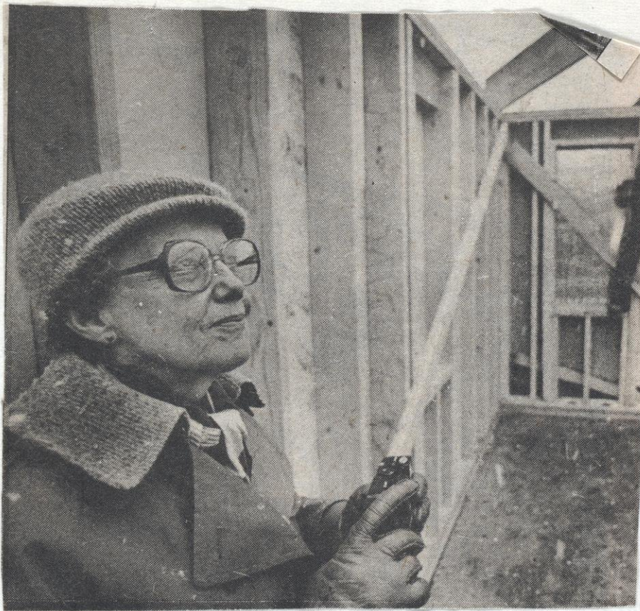
Barbara and Ted Arneson's house had to be demolished.
