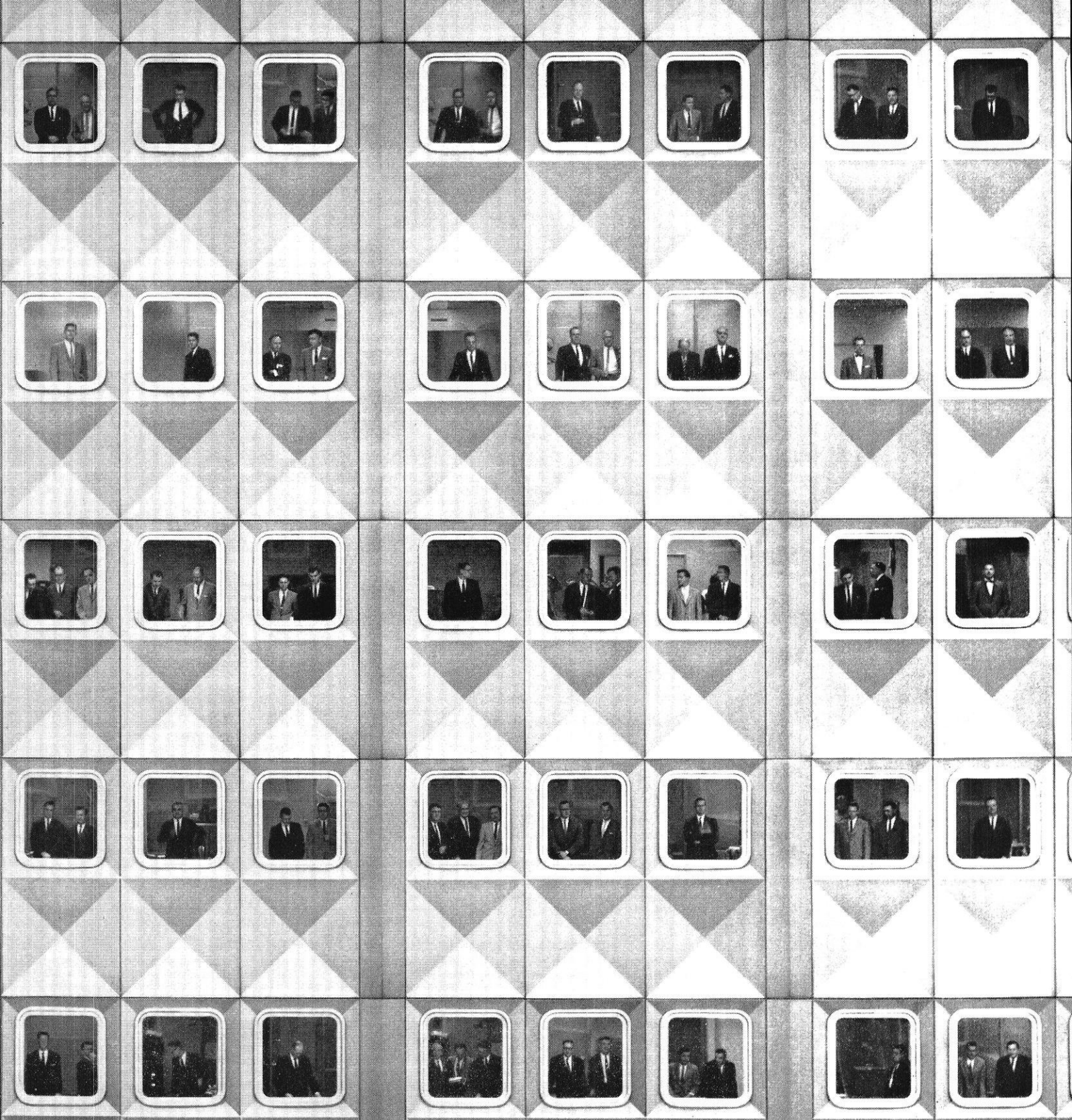
East wall of Alcoa's home office, Pittsburgh
