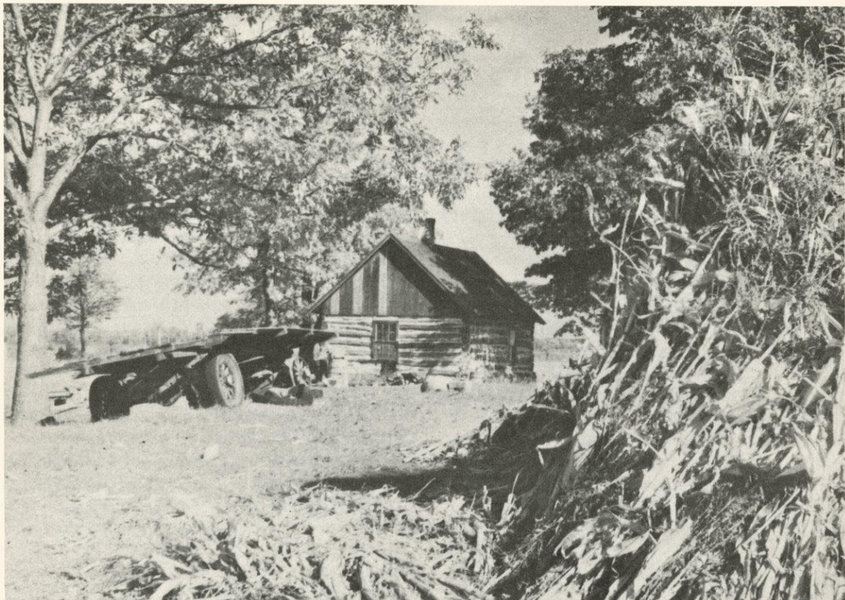
Log cabin still in use near Outagamie line
