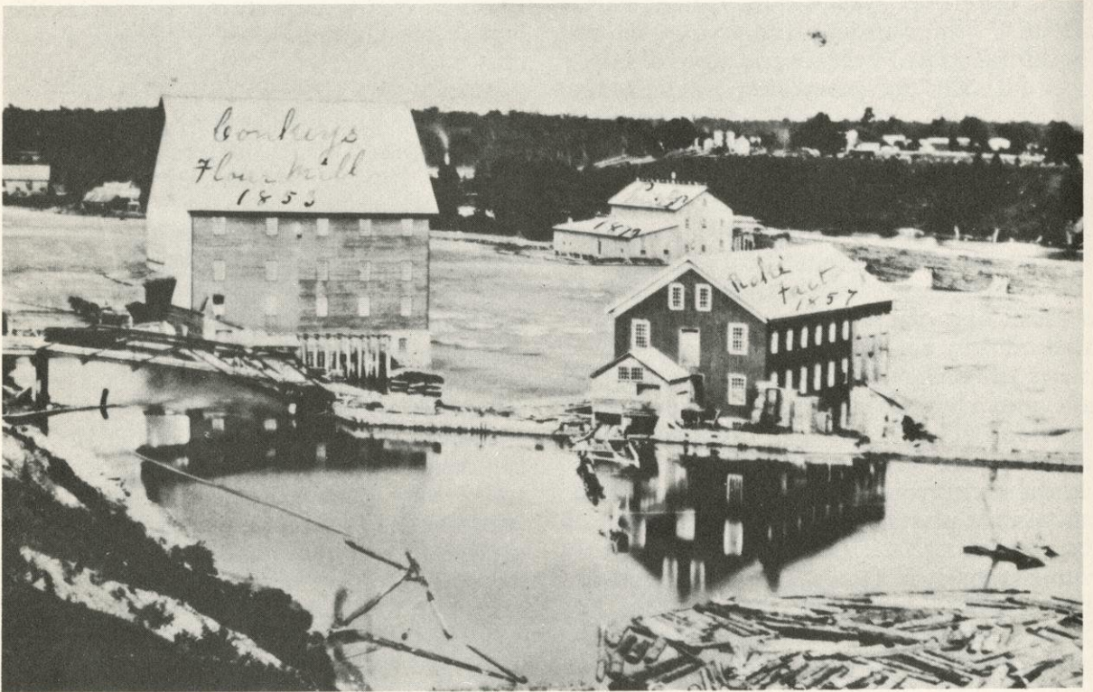
Early Industry—Conkey Flour Mill (1853) on the left; pulp mill in center background; Rake Factory (1857) at right.
