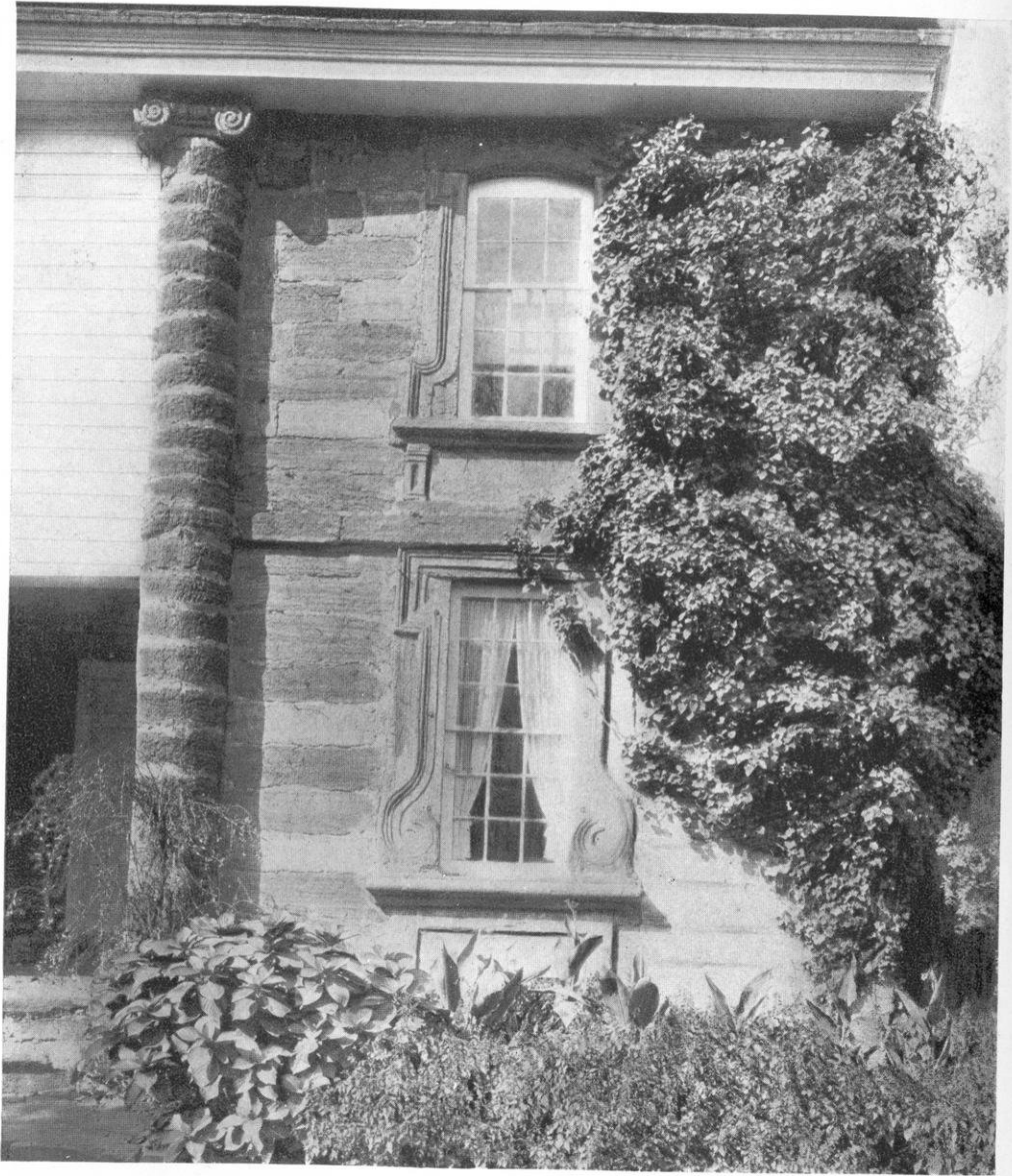
A DETAIL OF THE BARTRAM HOUSE, SHOW- ING EXTREMELY INTERESTING PILLAR OF CON- CRETE, WITH DORIC CAPITAL.
