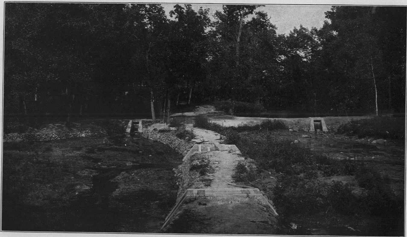
TROUT PONDS IN PROCESS OF CONSTRUCTION, WILD ROSE.
