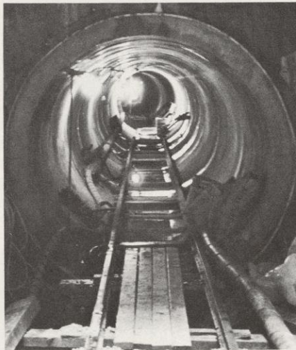
Inside a six-foot-diameter pipe in Milwaukee, 70 feet below ground. When completed, this multi-million-dollar project will separate all sanitary sewer lines from storm sewers so that Milwaukee's sewage plant won't be overloaded by every heavy thunderstorm. The construction is partially funded by the Wisconsin Fund. Photo by author.
