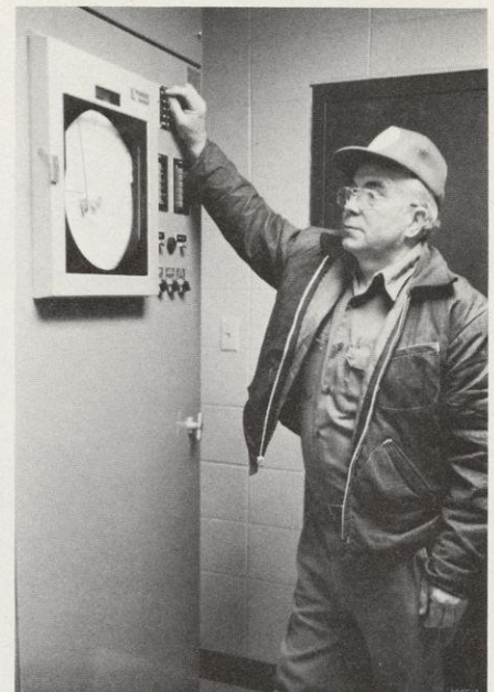
Plant operator Jim Palmer checks flowmeter that measures the volume of incoming sewage. The Orfordville plant treats 100,000 gallons daily. Photo by author
