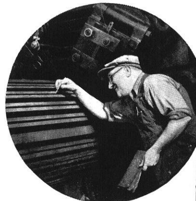
New Allis-Chalmers turbines add U.S. Industry's growing power.
