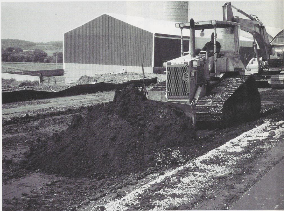
Spent foundry sands compact well and make an excellent fill in road bases and embankments.
