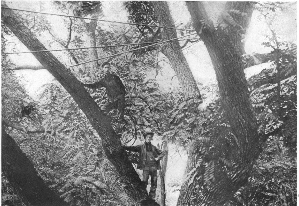
LIMBS OF TREES PROPERLY SUPPORTED BY IRON BARS HELD BY BOLTS AND WASHERS, INSTEAD OF BANDS AROUND THE BRANCHES.
