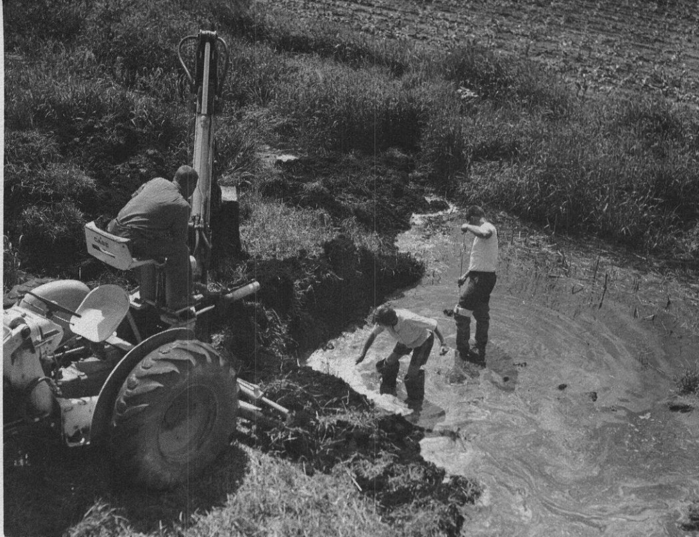
Probing in the excavation pit.
