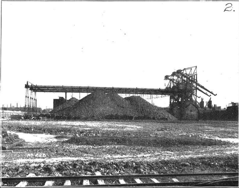
Coal Handling Machinery at Milwaukee Plant.
