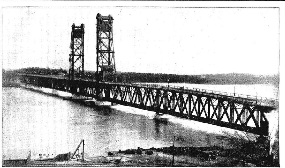
HIGHWAY AND RAILROAD BRIDGE AT BATH, MAINE PIERS AND APPROACHES CONSTRUCTED BY THE FOUNDATION COMPANY
