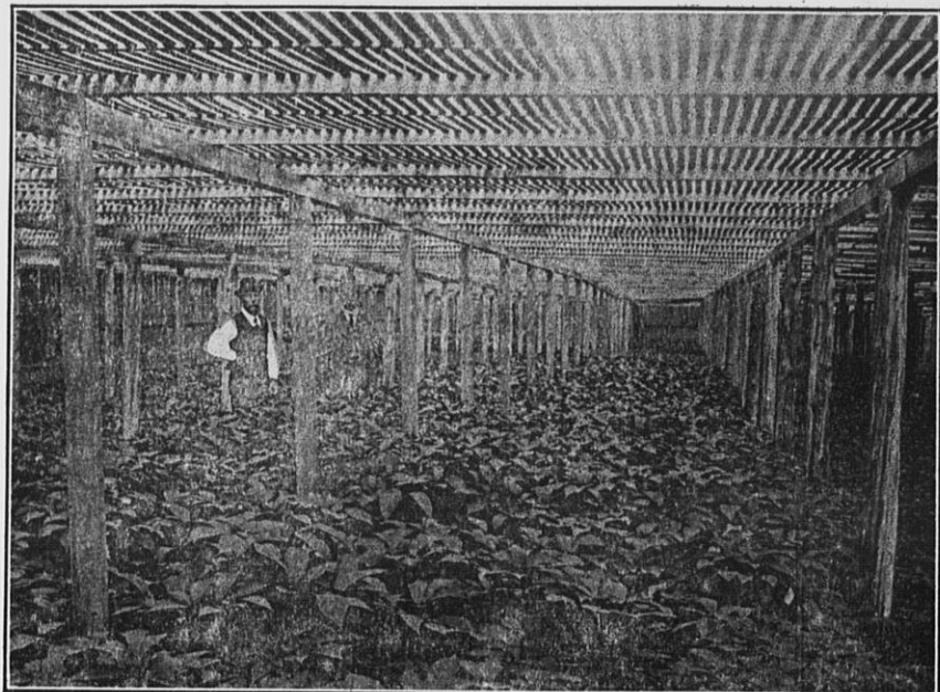
FIG. 1.—The above illustration is a reproduction of a photograph taken in one of our gardens showing thousands of ginseng plants as they appeared in their fourth year's growth. It also shows construction of the shade arbor, the roof of which is made of plaster lath with \frac{1}{2} inch space between the lath.
