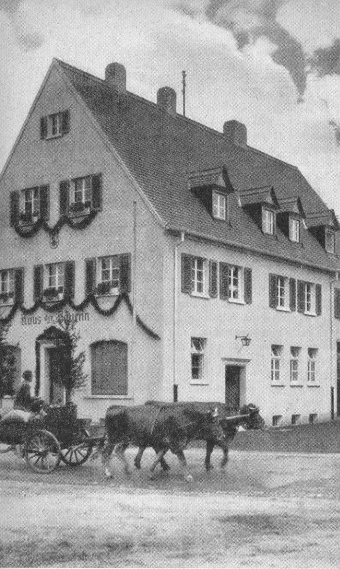
Modern labor-saving devices installed in seven newly-built community houses are making life easier, pleasanter in Bavaria. New projects have proved tremendously popular — and inspired many communities to follow suit.
