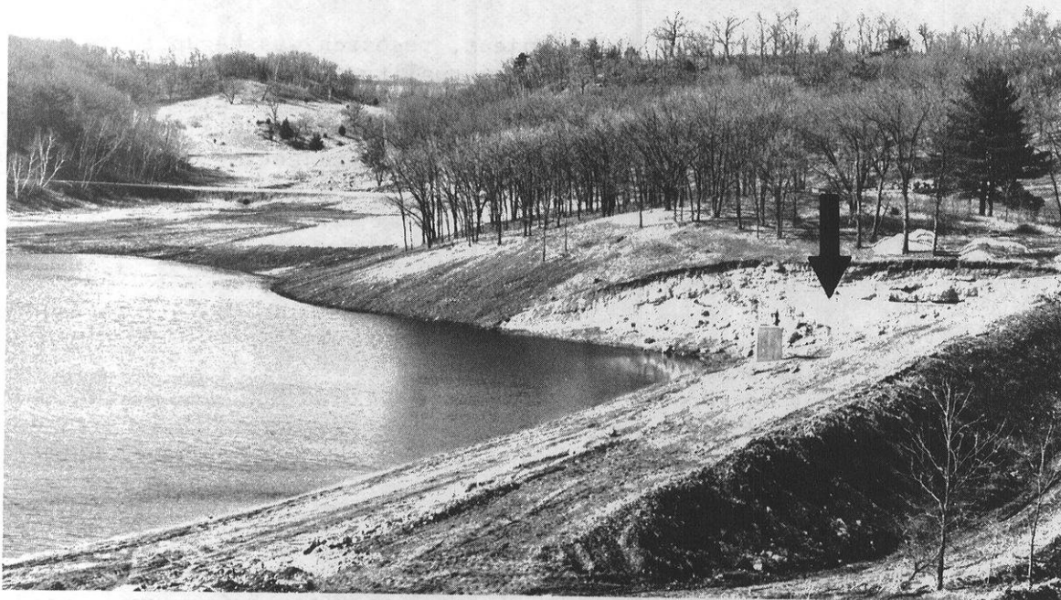
The earthen dike and the concrete spillway. The arrow indicates the rectangular notch which allows for the continuous discharge of water.
