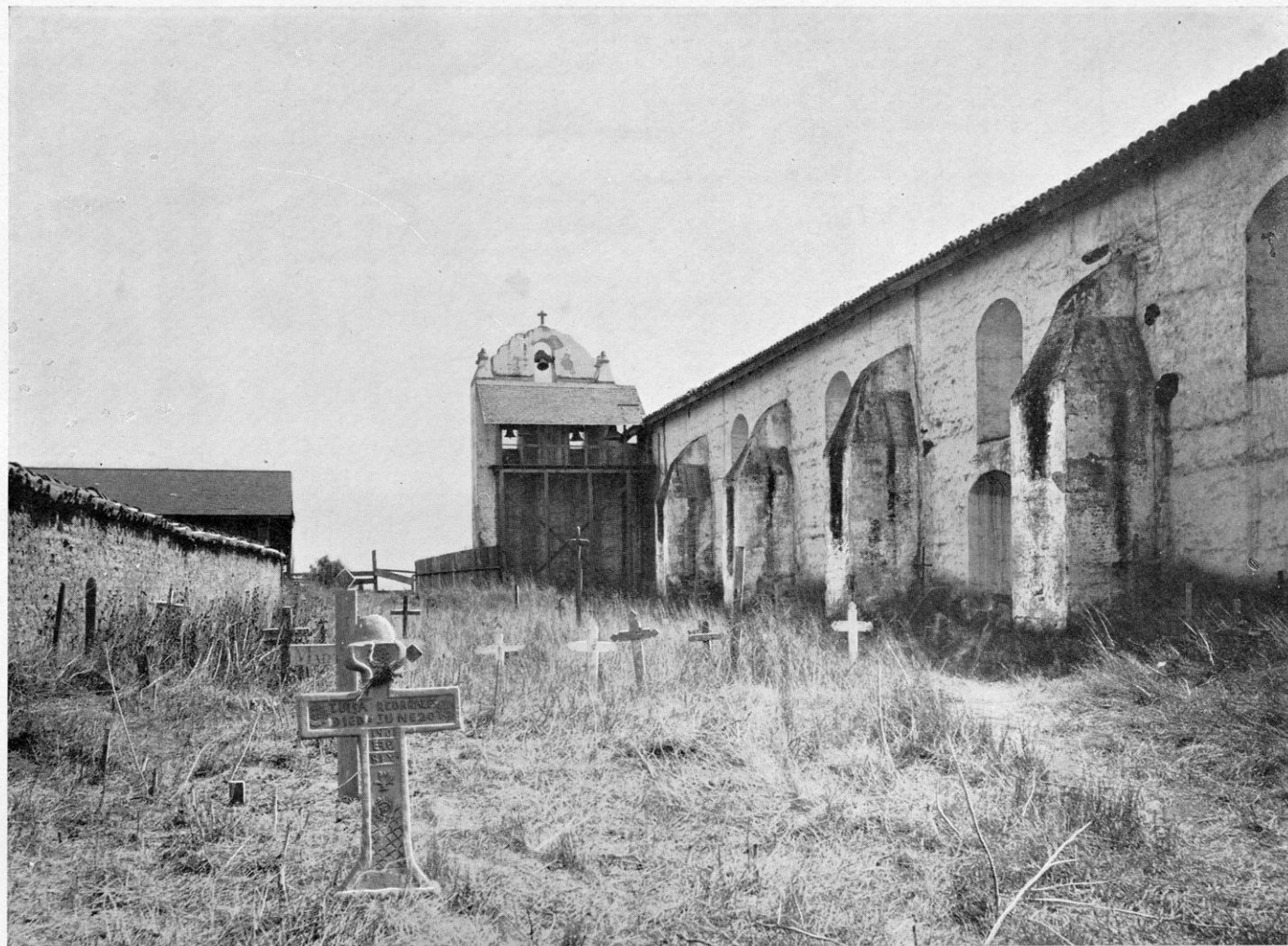
Figure VI. Santa Inez : side wall showing buttress construction
