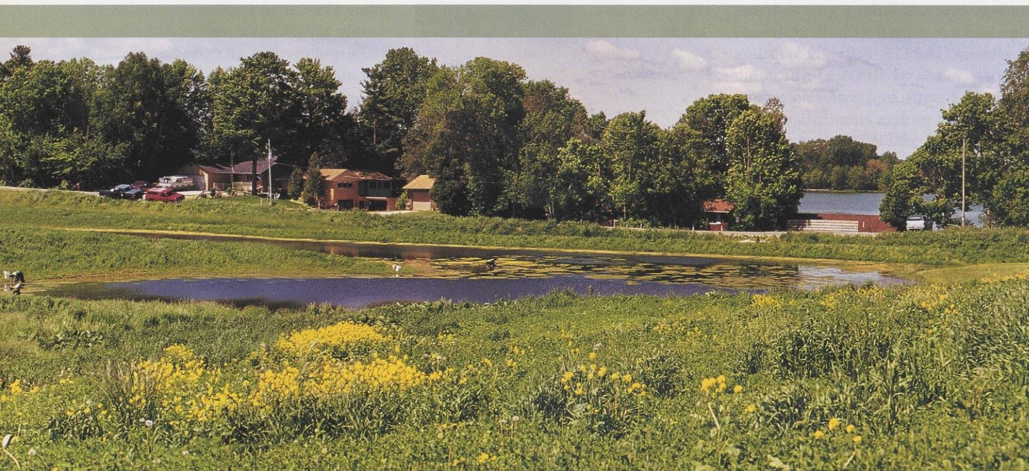
Viewed from the farmhouse, you can see how the bermed detention pond allows stormwater nutrients to settle and soak in before cleaner water flows into English Lake.
