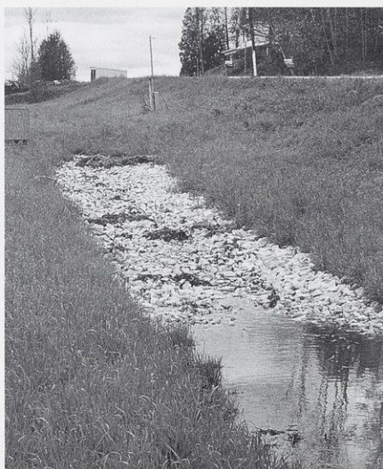
After stormwater settles in the basin, a crushed rock outlet filters additional solids before water flows into English Lake. Instruments in the monitoring shed measure the amount of pollution removed by the basin.
