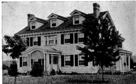
Walls finished with Cabot's Old Virginia White, roof finished with Green Cabot's Creosote Stain. "We are using the same stains on other houses with equally satisfactory results."—Herbert Feltz, Architect, Indianapolis.
