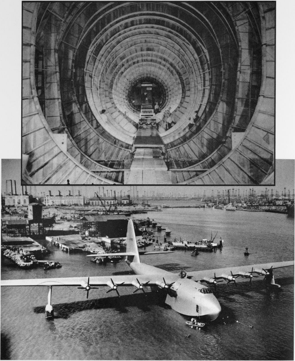
Figure 10.3. Hughes H-4 Hercules giant flying boat, with detail of fuselage interior under construction. National Air and Space Museum, Smithsonian Institution (SI neg. nos. 79-5026 and 71-142-12).
