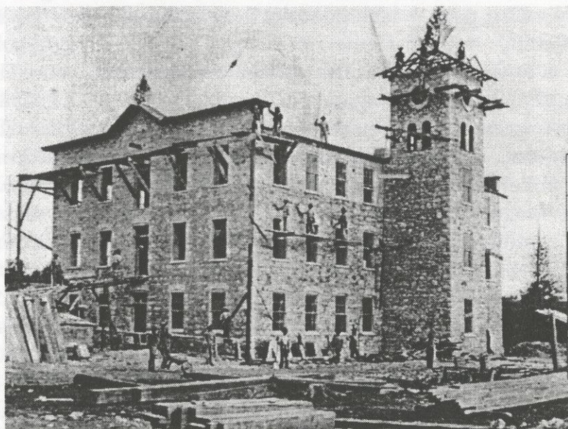
Woolen Mill, under construction, 1880.
