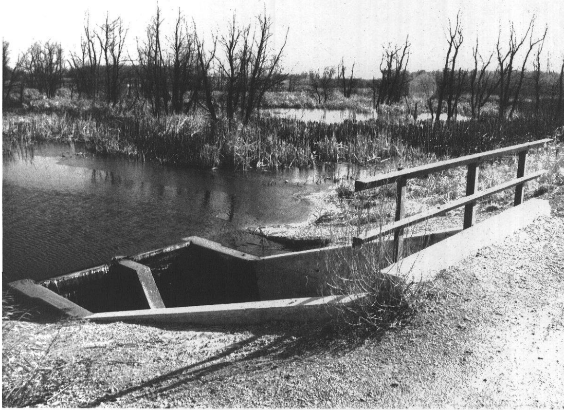
Eldorado Marsh control structure. Note that outer sections of the side abutments act as part of the spillway.
