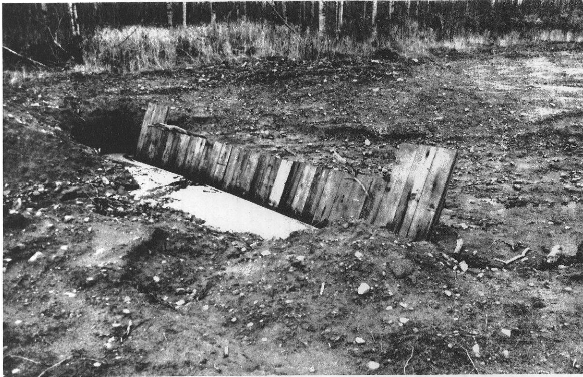
Beginning of wooden spillway installation, Antigo District
