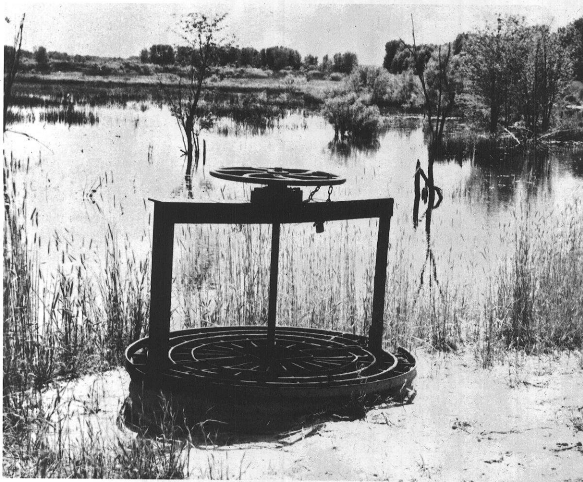
Tin whistle with sliding gate and handwheel control, Mead Wildlife Area.
