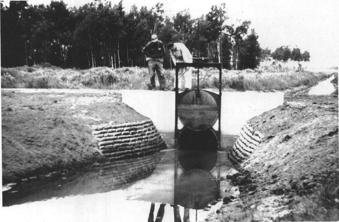
Sliding steel gate used on Crex Meadows Wildlife Area for impoundment water level control. The handwheel on the top frame turns a threaded shaft attached to the gate and this moves the gate up or down.
