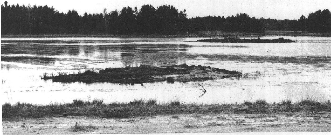
"Push-up" islands constructed by bulldozer (Black River Falls Districts).
