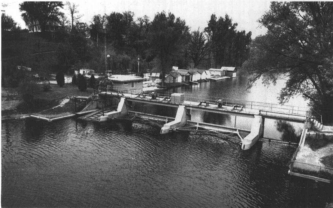
Horicon Marsh dam. Note radial gates and stoplog bays.
