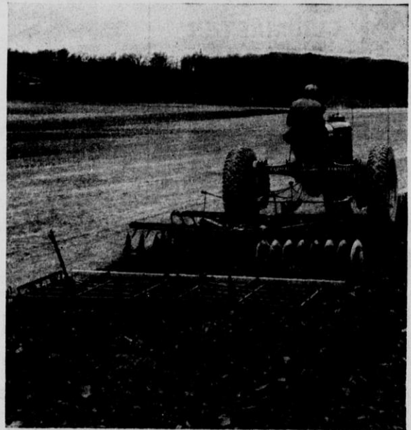
Above: Drilling moves along fast with a McCormick-Deering Grain Drill and Farmall 20 Tractor on the job. Right: A good job of disking and harrowing. The disk is an 8-foot McCormick-Deering with a 2-section McCormick-Deering Peg-Tooth Harrow pulled behind.
