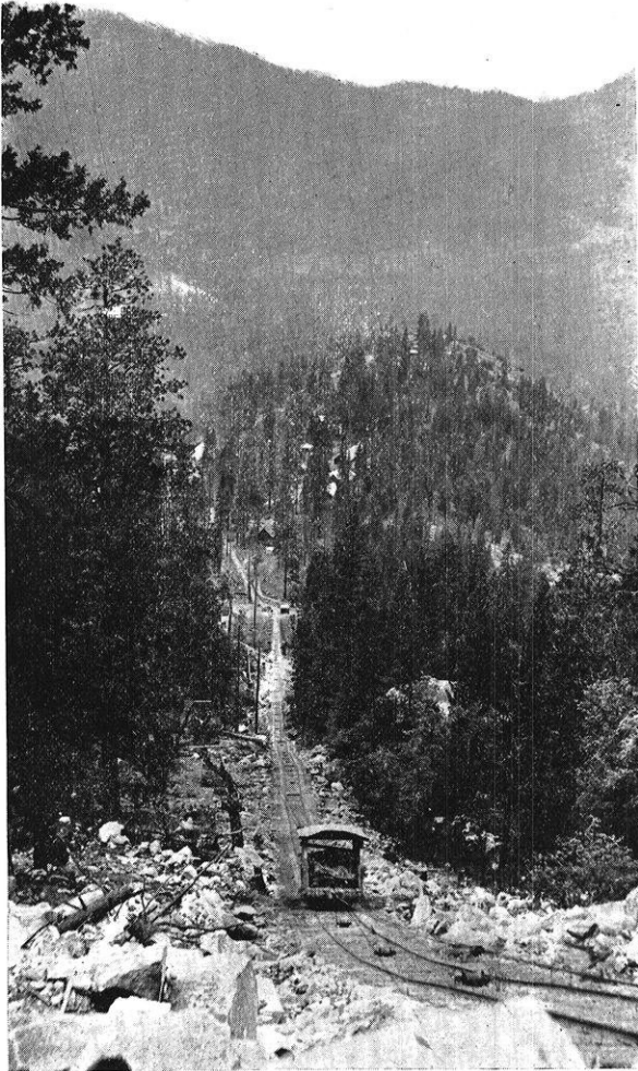
FIG. 2.—Hoist No. 1 Leading from Cascada to the Basin Maximum Gradient 85 Per Cent.
