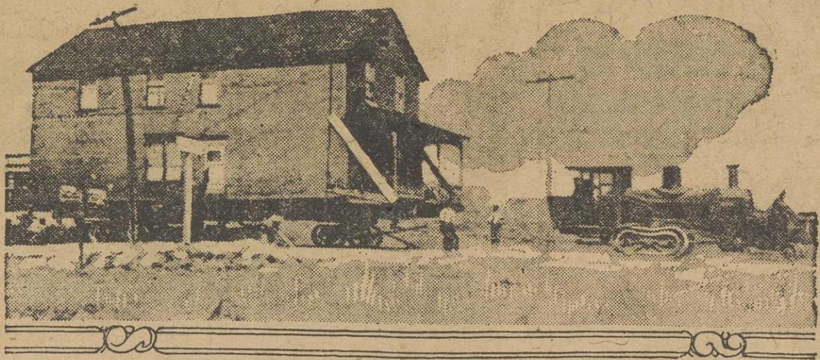
Steam caterpillar tractor, built for log hauling, pulling house to new foundation.
