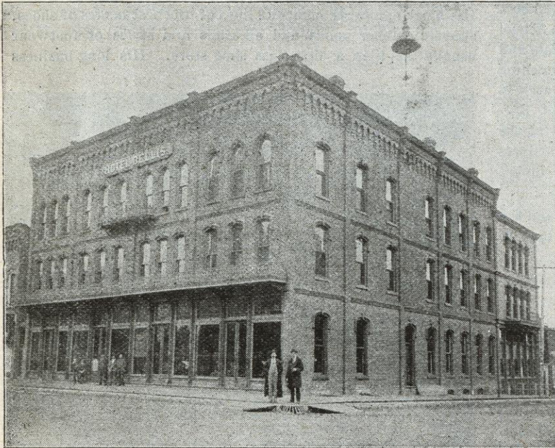
THE HOTEL BELLIS, CORNER OF THIRD AND SCOTT STREETS.
