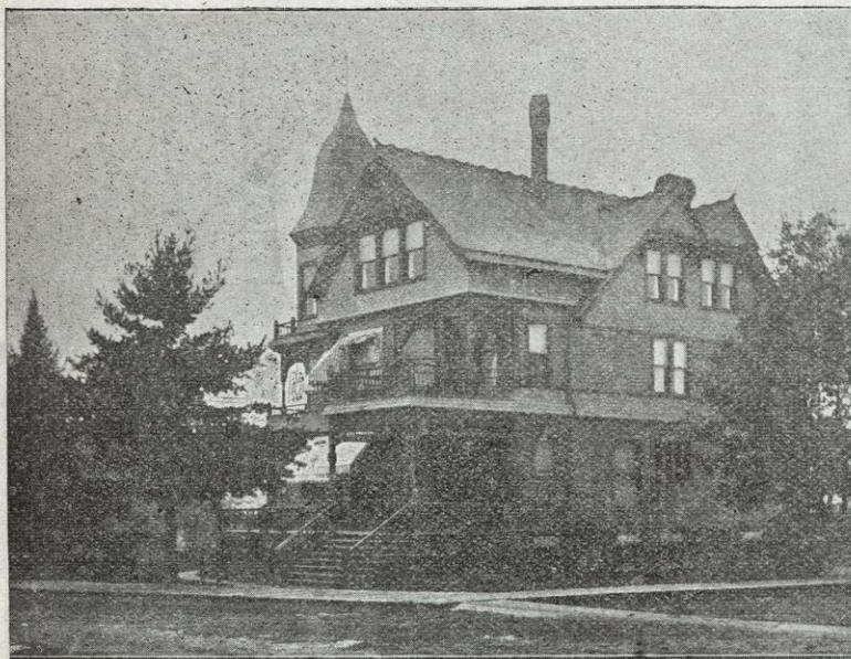
RESIDENCE OF HON. H. M. THOMPSON, MOSINEE.
