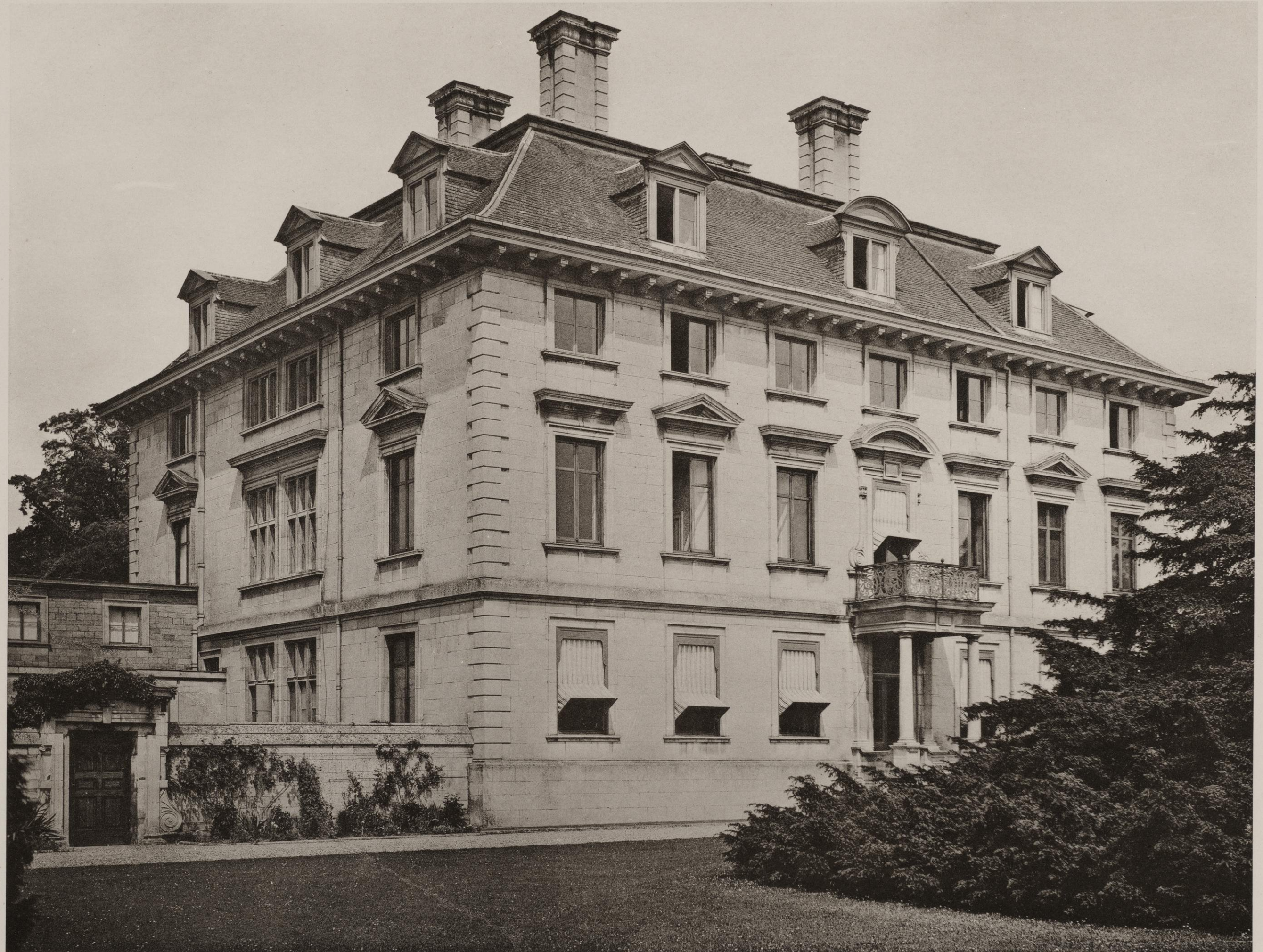
THORPE HALL, PETERBOROUGH. THE SOUTH FRONT.
