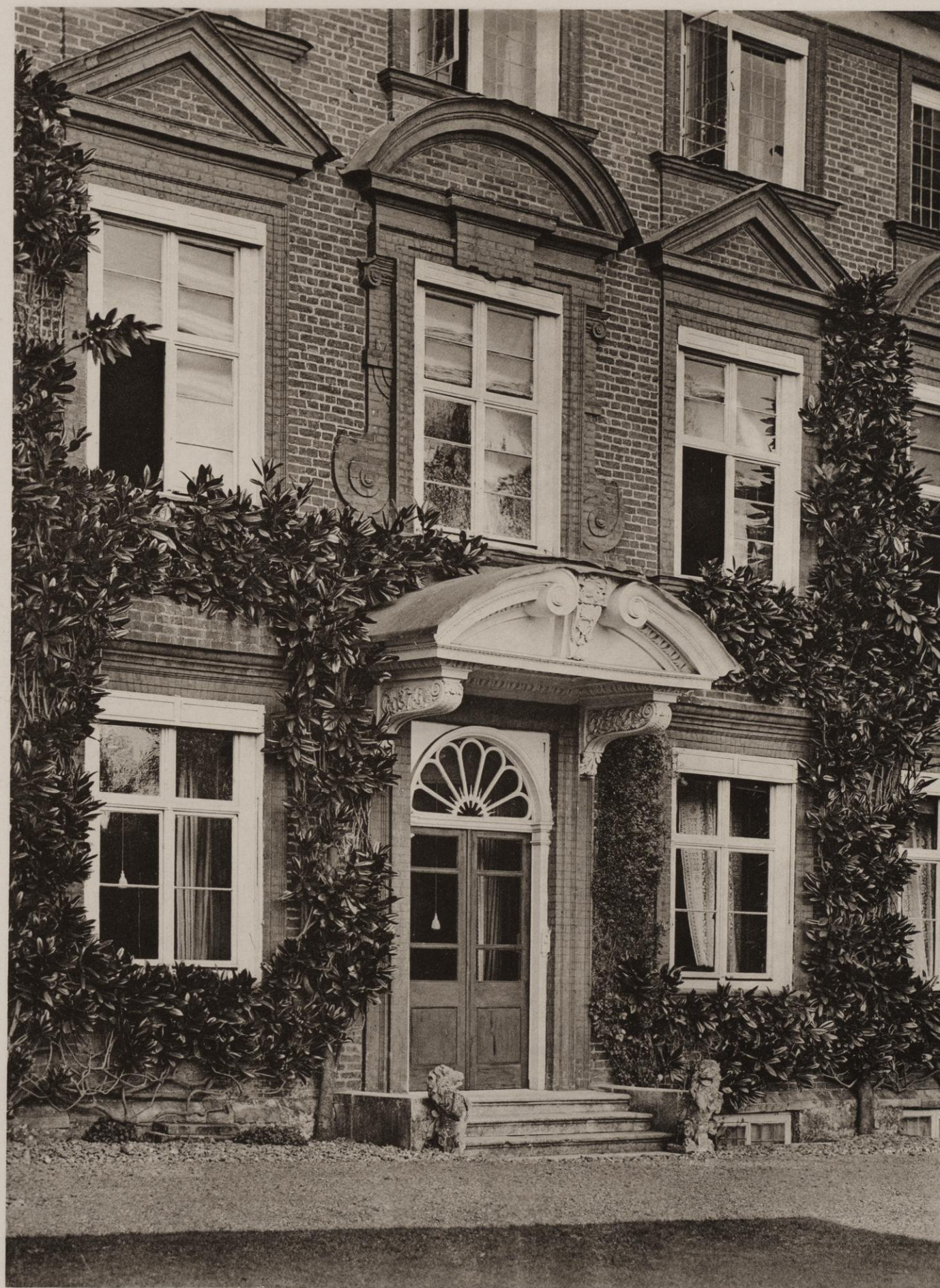
TYTTENHANGER, HERTS. ENTRANCE, GARDEN FRONT.
