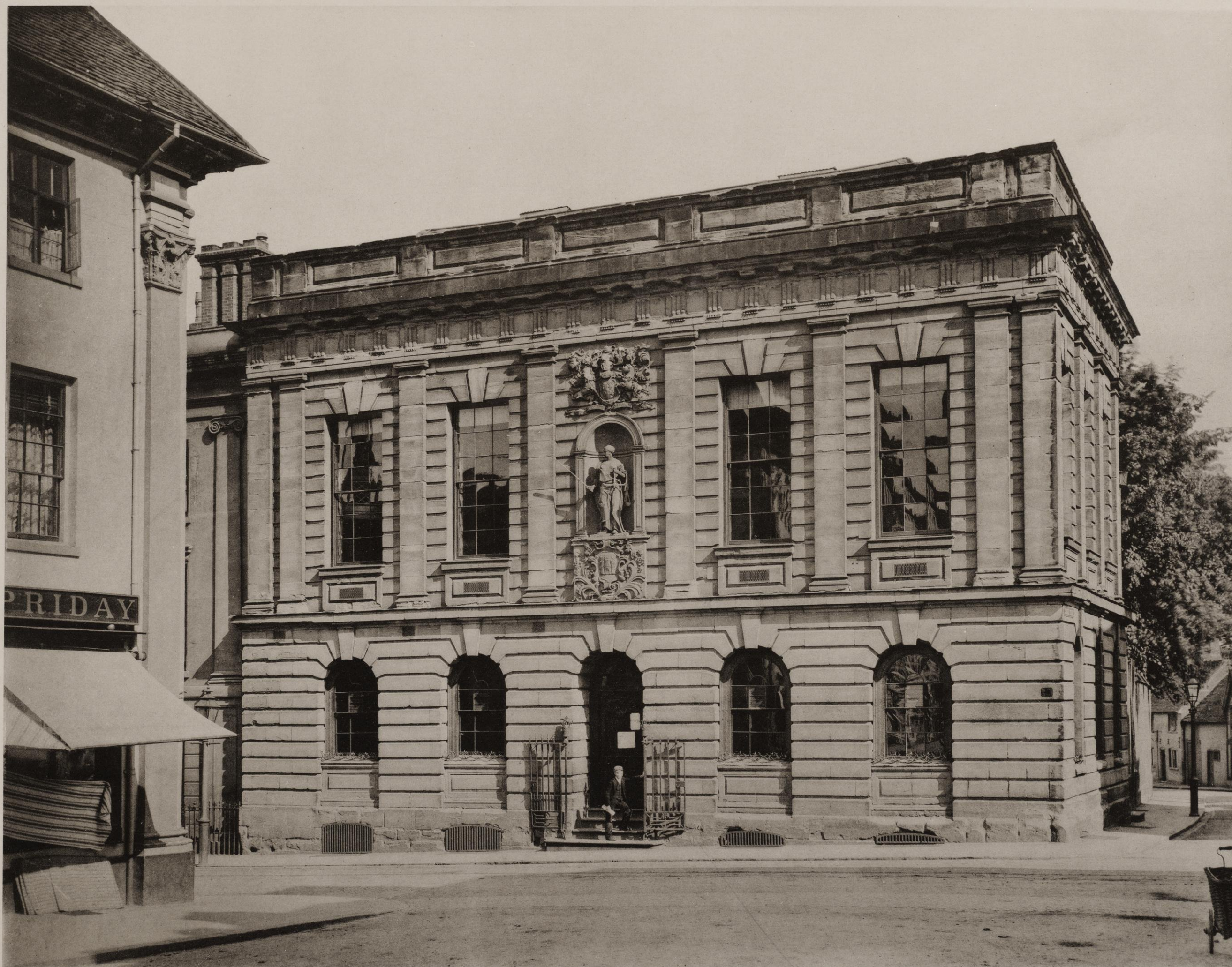
THE TOWN HALL, WARWICK.
