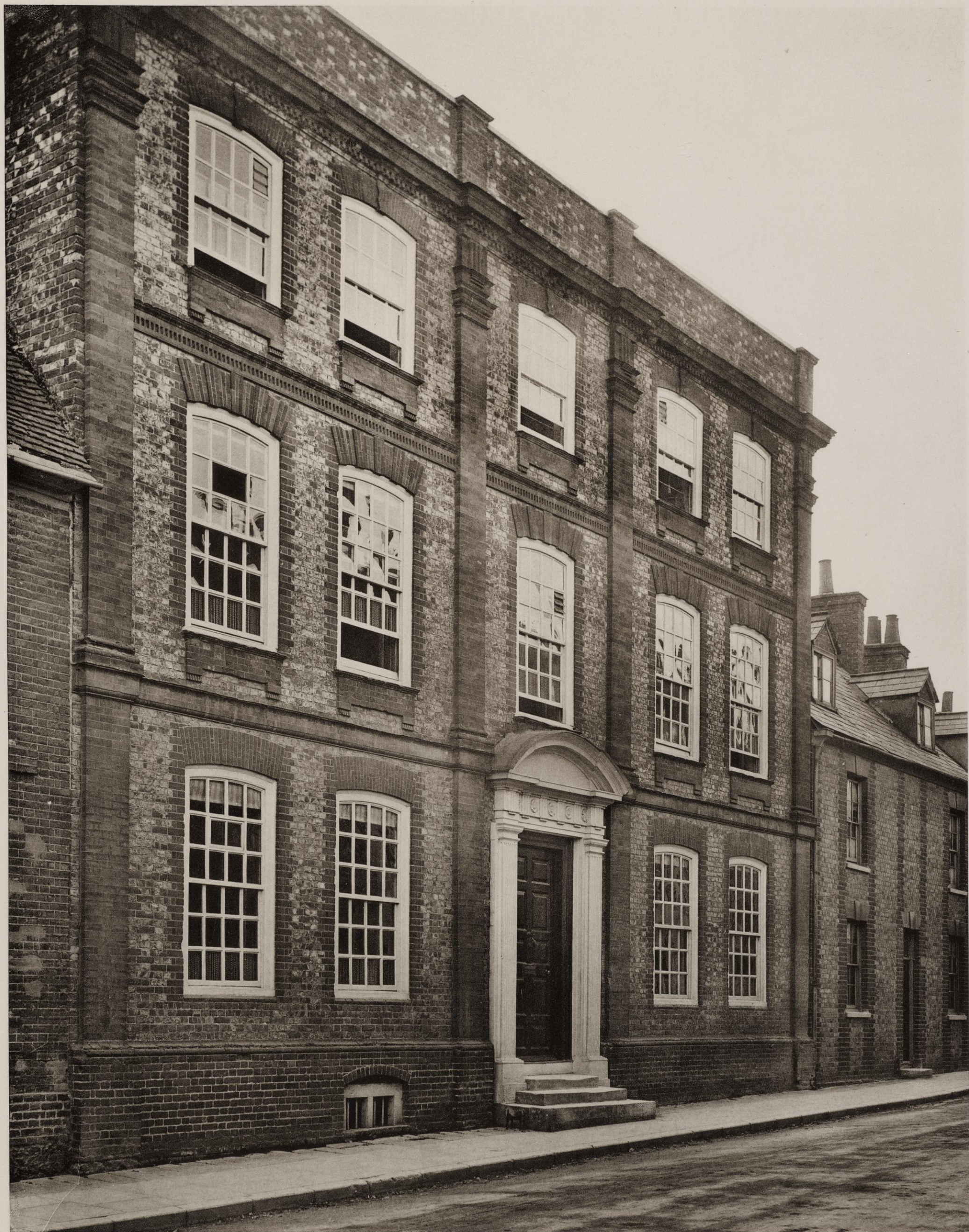
HOUSE IN HIGH STREET, WALLINGFORD.
