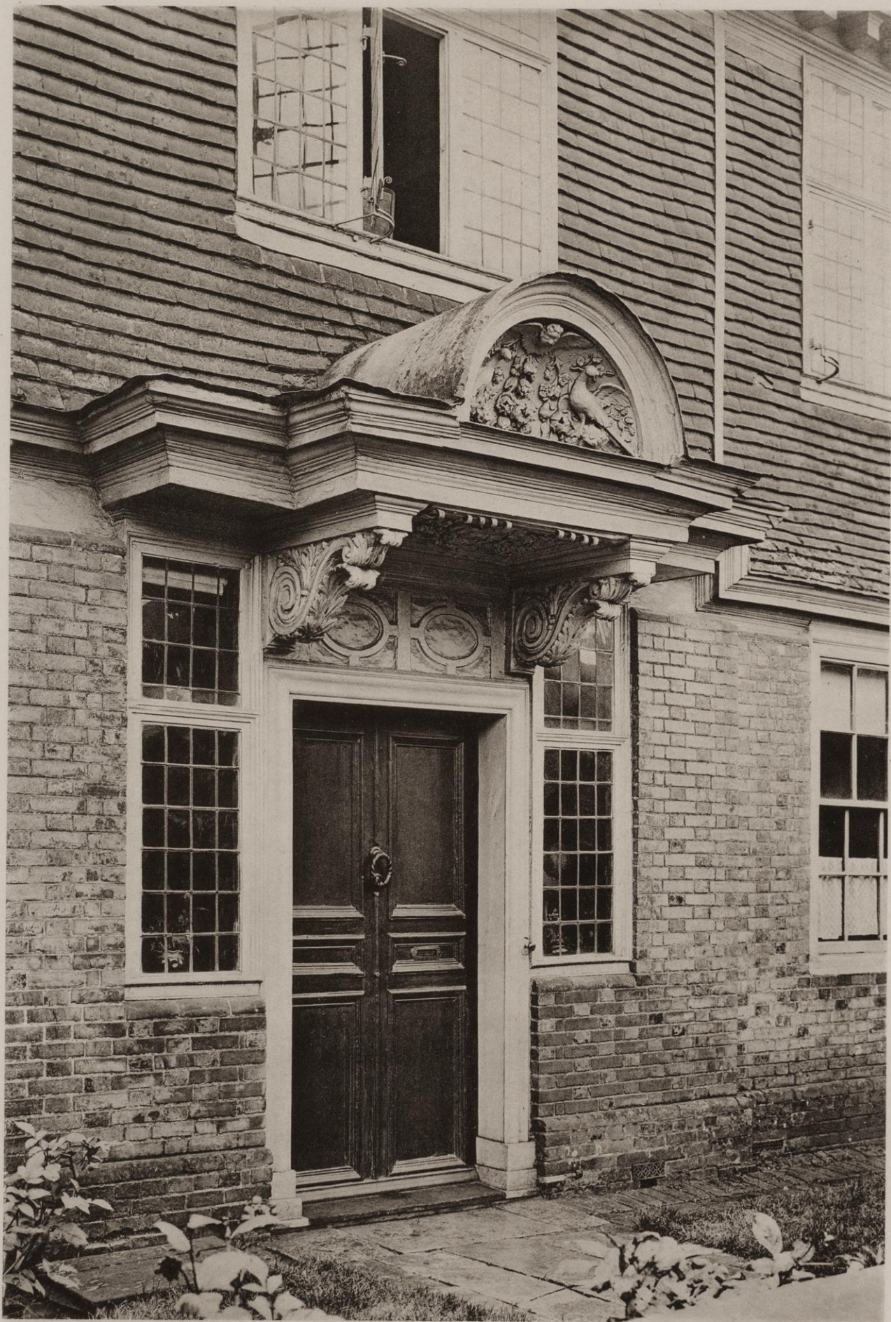
HOUSE AT BURWASH. DOORWAY.
