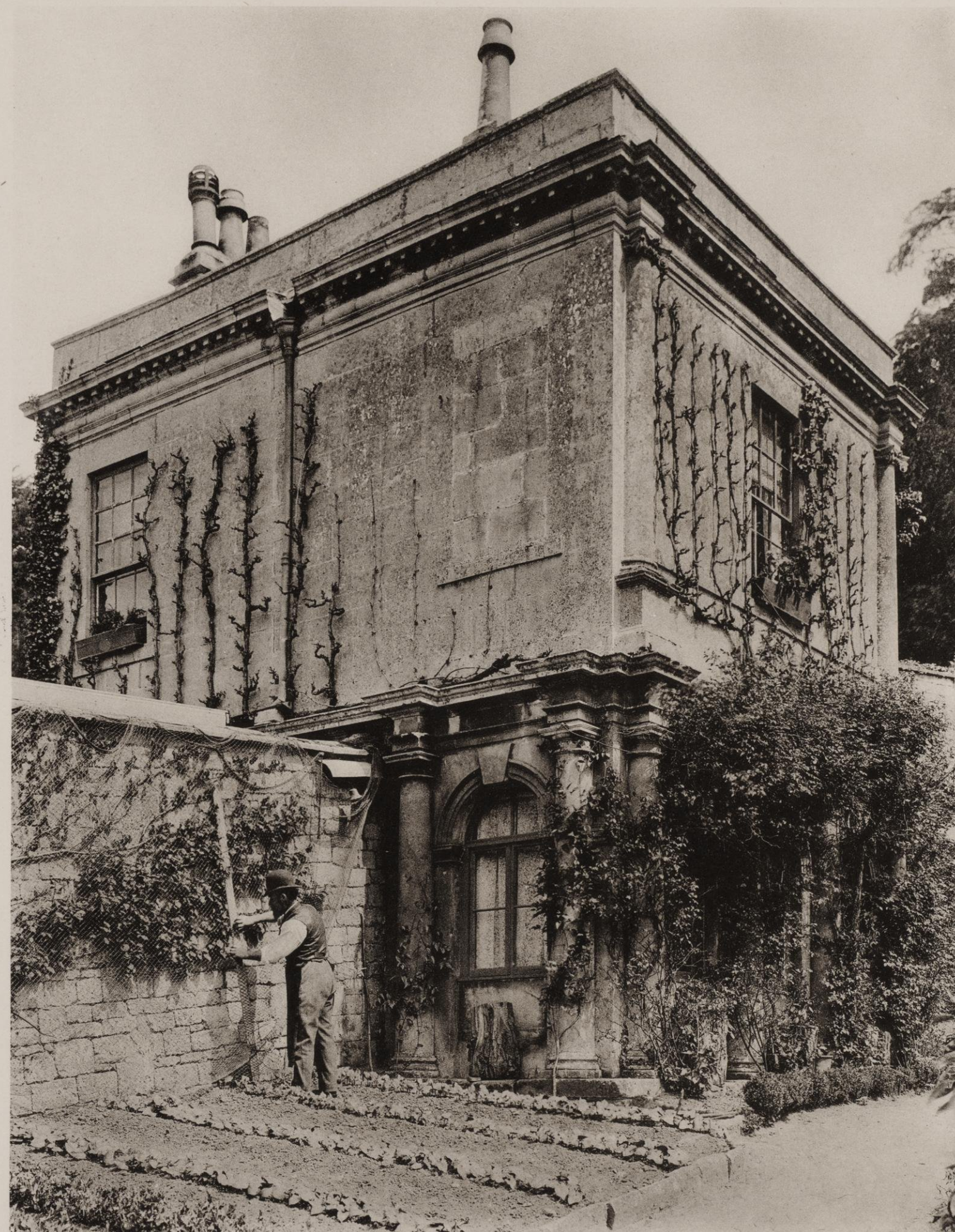
GARDENER'S LODGE, WIDCOMBE, BATH.
