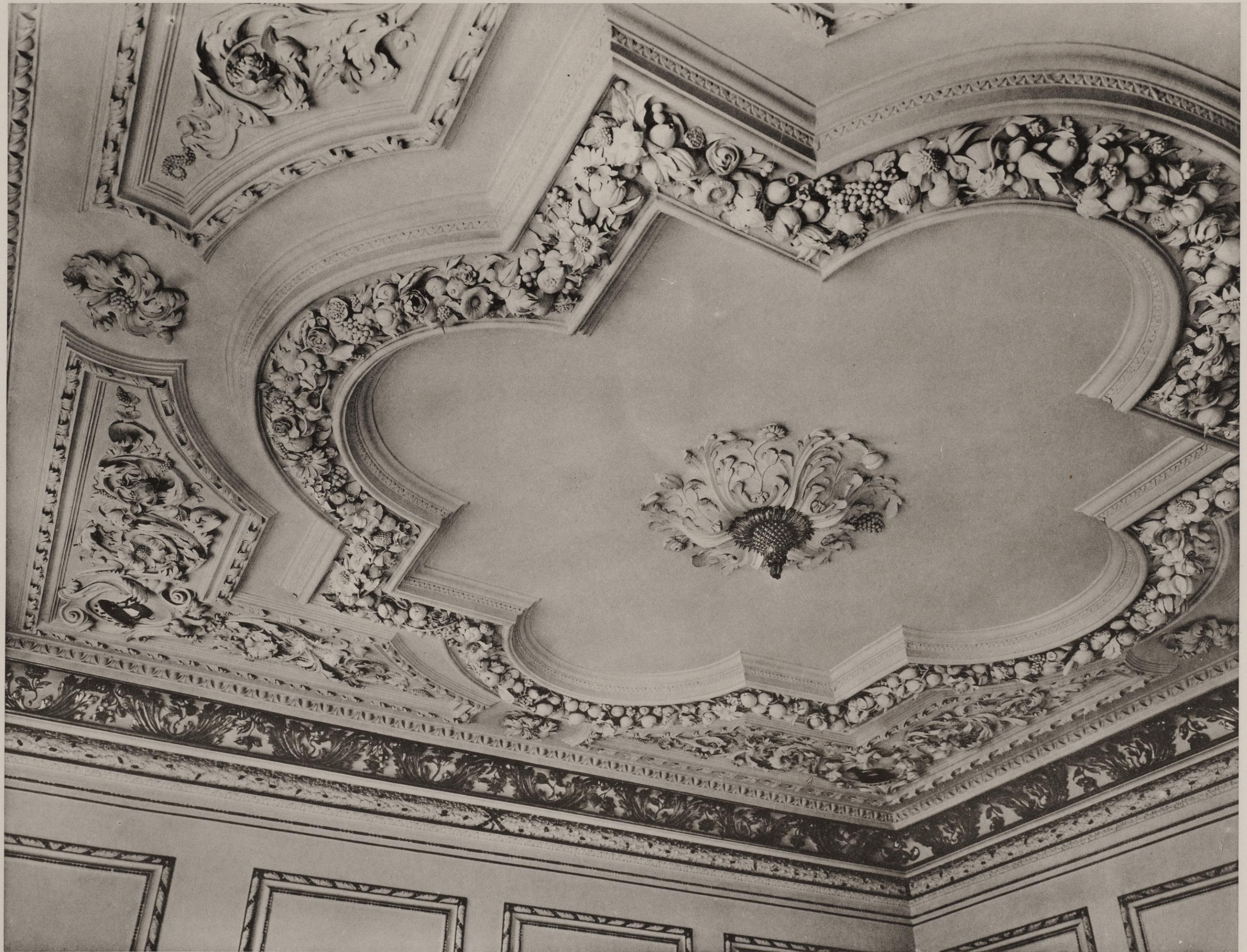
BELTON HOUSE, GRANTHAM. CEILING OF THE STAIRCASE.
