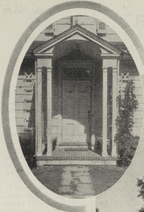
The illustration above shows the door of this attractive house in detail. It brings out strikingly the clean cut mouldings that are used and that do much to make the house distinctive. The architects have used simple inexpensive materials throughout, and through good proportions have attained excellent results
