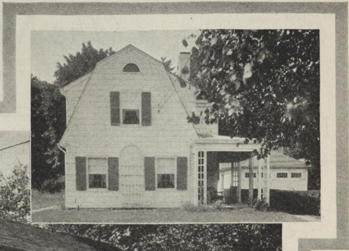
The illustration at the right shows the porch end of the plan, ideally located for this particular spot with the big tree for shade. Porch curtains the color of the shutters would give a unifying effect, and also at times make the porch cosier and more livable
