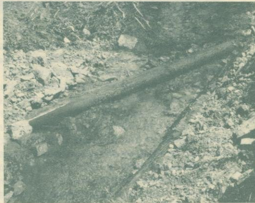
An upstream view of a "cross-log and revetment" device placed in Camp Creek. This structure creates a scour pool as water drops over the cross-log placed at an angle to the flow. Water is diverted in direction toward the bank where the revetment log has been placed. This log provides hiding cover for trout in the pool and also protects the bank from erosion.
