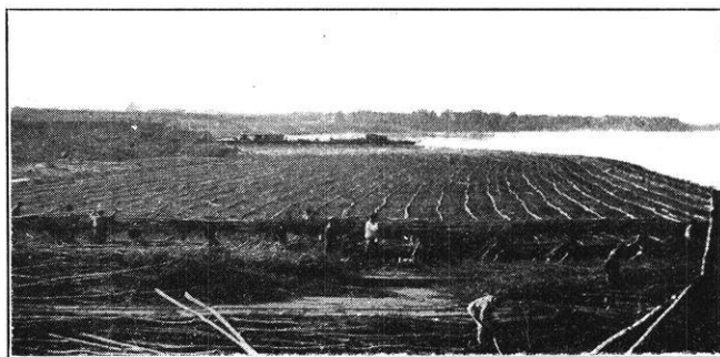
FIG. 2. POLE CRIBS BUILT ON TOP OF MAT TO HOLD STONES IN PLACE
