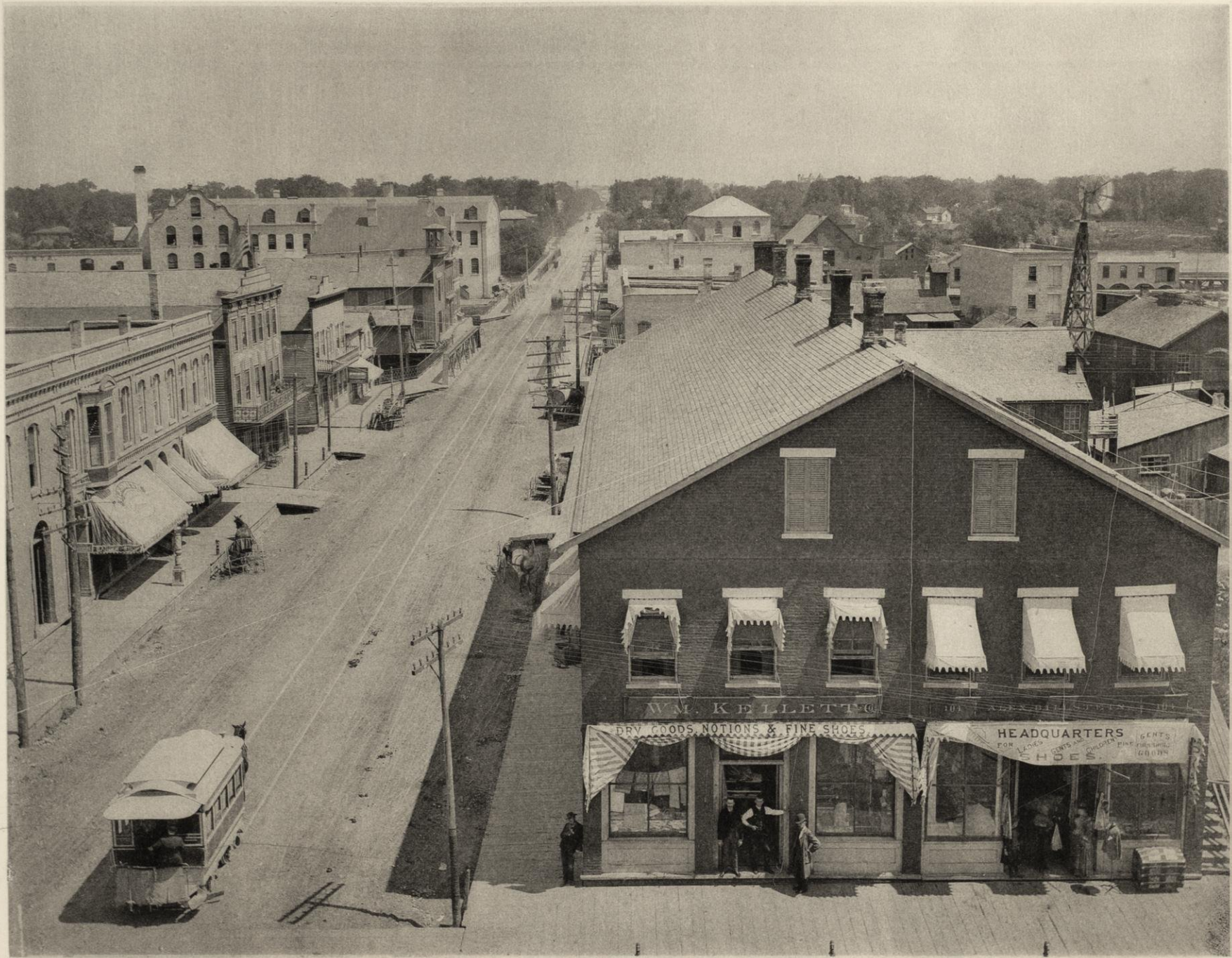
NEENAH—LOOKING NORTH FROM TOP OF RUSSELL HOUSE.
