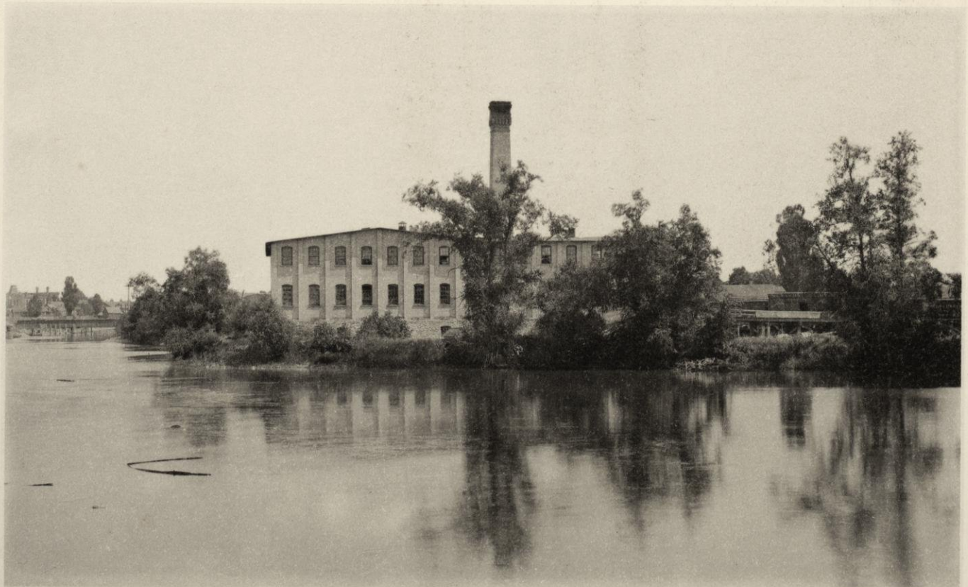
MENASHA—CANAL NEAR THE LOCKS, AND PAPER MILL OF GEO. A. WHITING.
