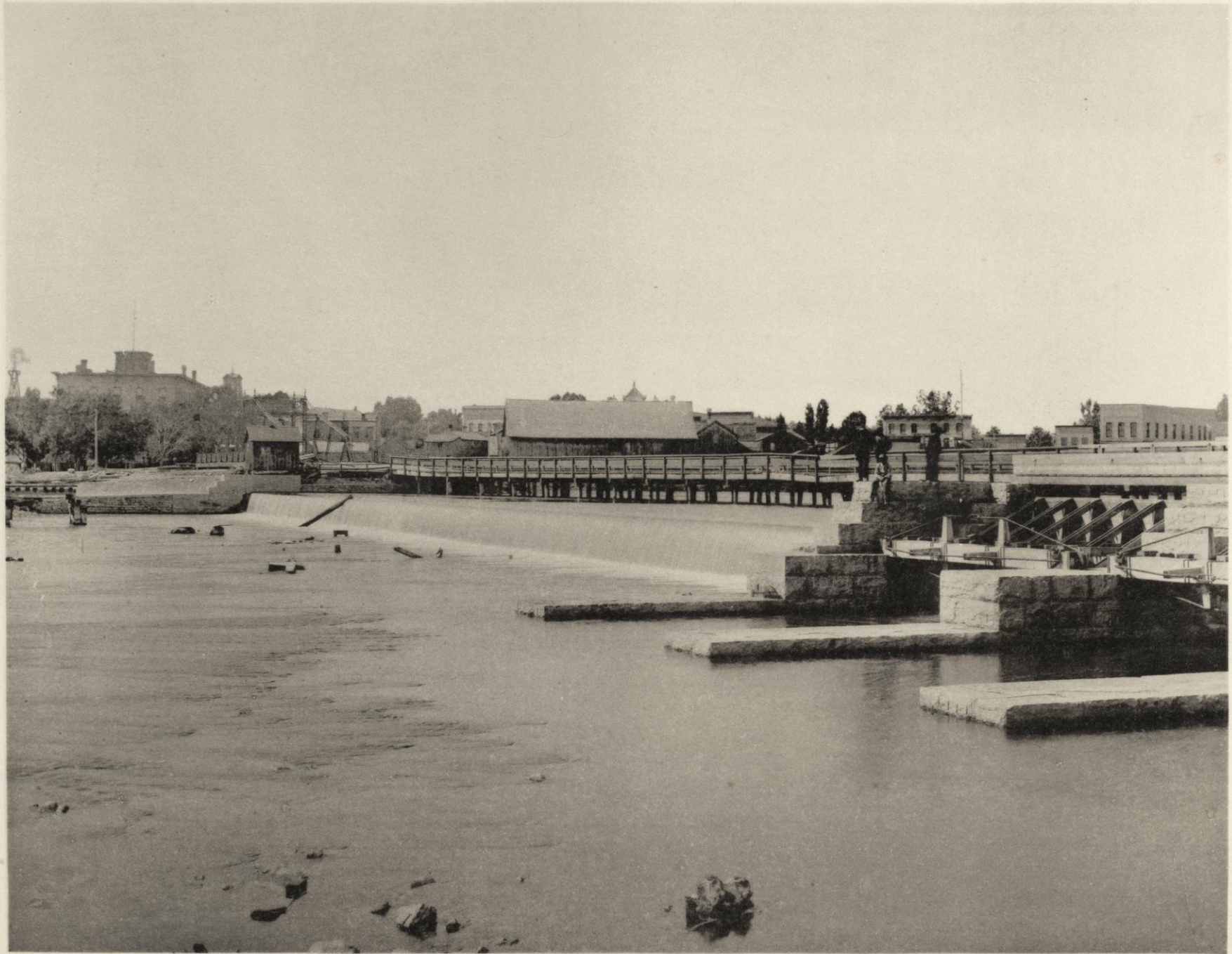
MENASHA—FROM SOUTH END OF DAM, LOOKING NORTH.
