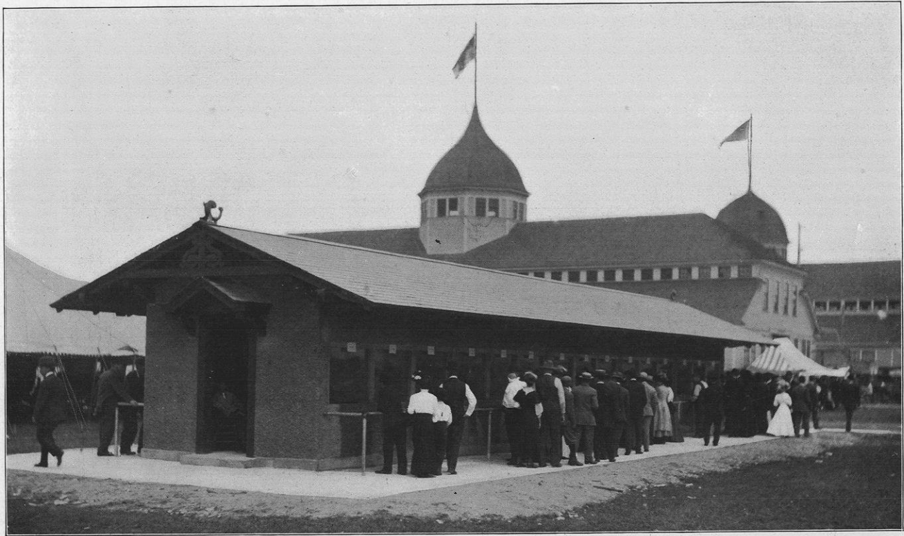
THE FISH EXHIBIT BUILDING.
