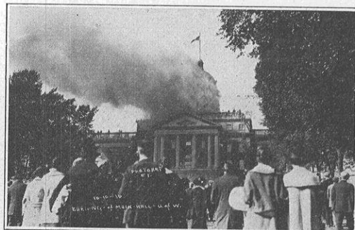
BASCOM HALL FIRE, 1916
