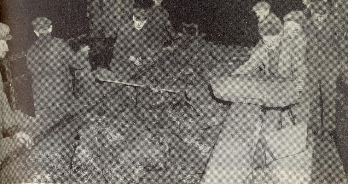
Surface workers pick stones out of coal as it comes from the washer on its way to be loaded into railroad cars at the Friedrich Krupp Hanover coal mine in Bochum, near Essen. (Photographs are by Al Byers, JEIA)
