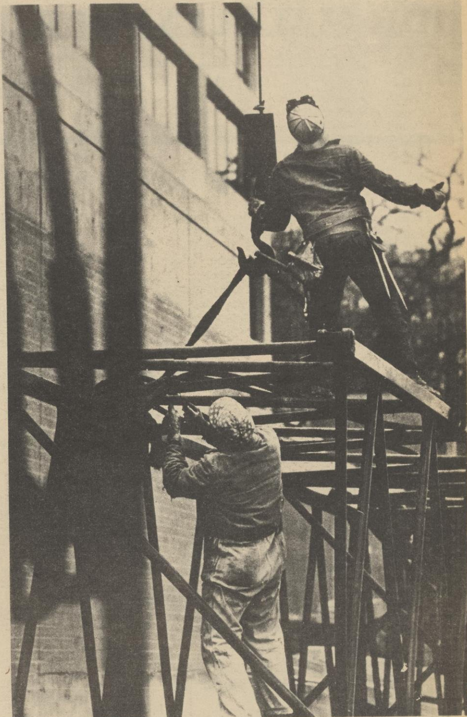
CONSTRUCTION WORKERS PREPARE an extension for the crane boom used at the Undergraduate Library now under construction at 600 N. Park St. The additional height is necessary to lift special concrete slabs for the building's windows. Cardinal photo by Michael Mally
